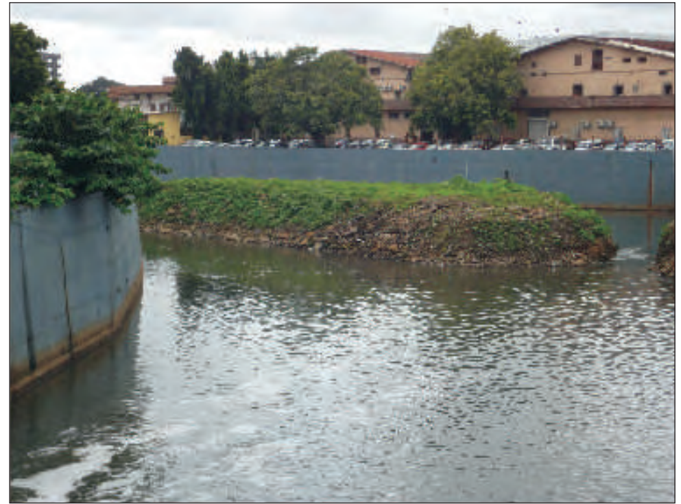
Figure 4.11- Concrete retaining walls have robbed the river of its banks. Photo courtesy: ORF Mumbai
