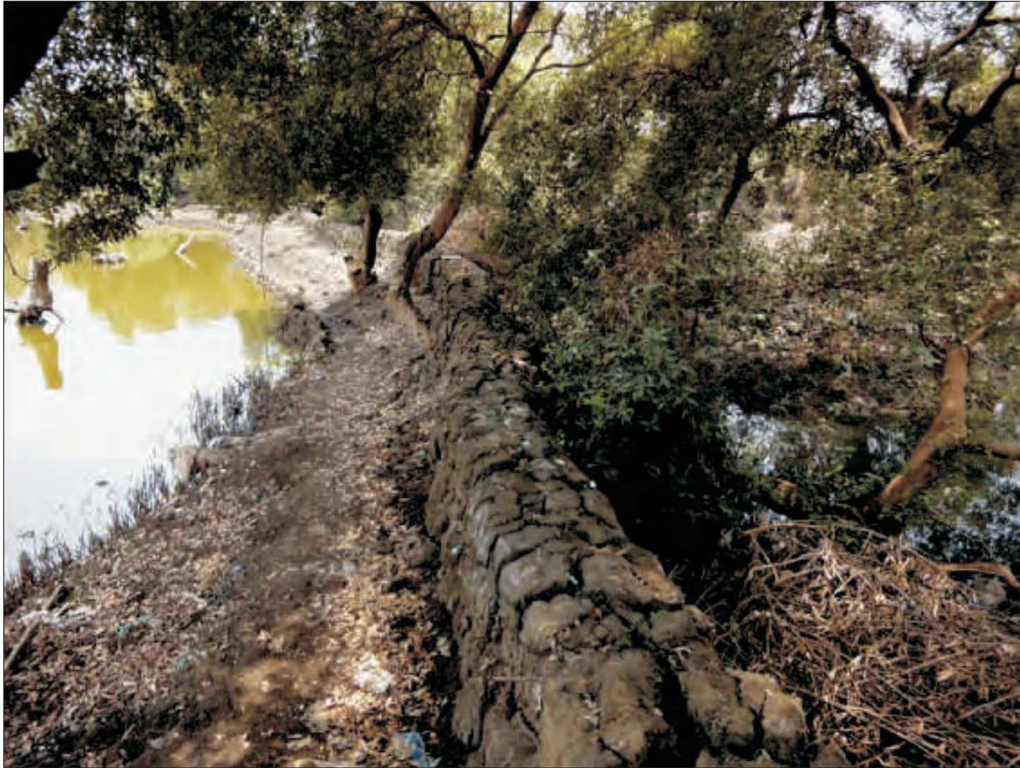
Figure 5.1- Clay embankment built to create fish farms inside the mangrove forest trapping estuarine waters during high tide. In this image, the difference in water levels on either sides of the banks is clearly visible. Photo courtesy: ORF Mumbai
