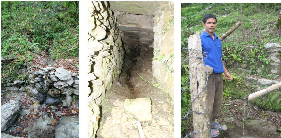
Springs are drying rapidly at all the locations of the hydropower project sites across the state due to high intensity explosions in the tunnels, road construction etc.
