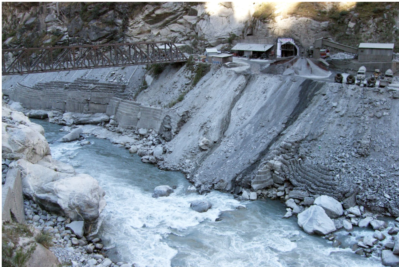
3. Photo 3 showing how the muck is flowing into the Sutlej river. Photo taken a few km downstream from the dam site on Nov 10 2010
