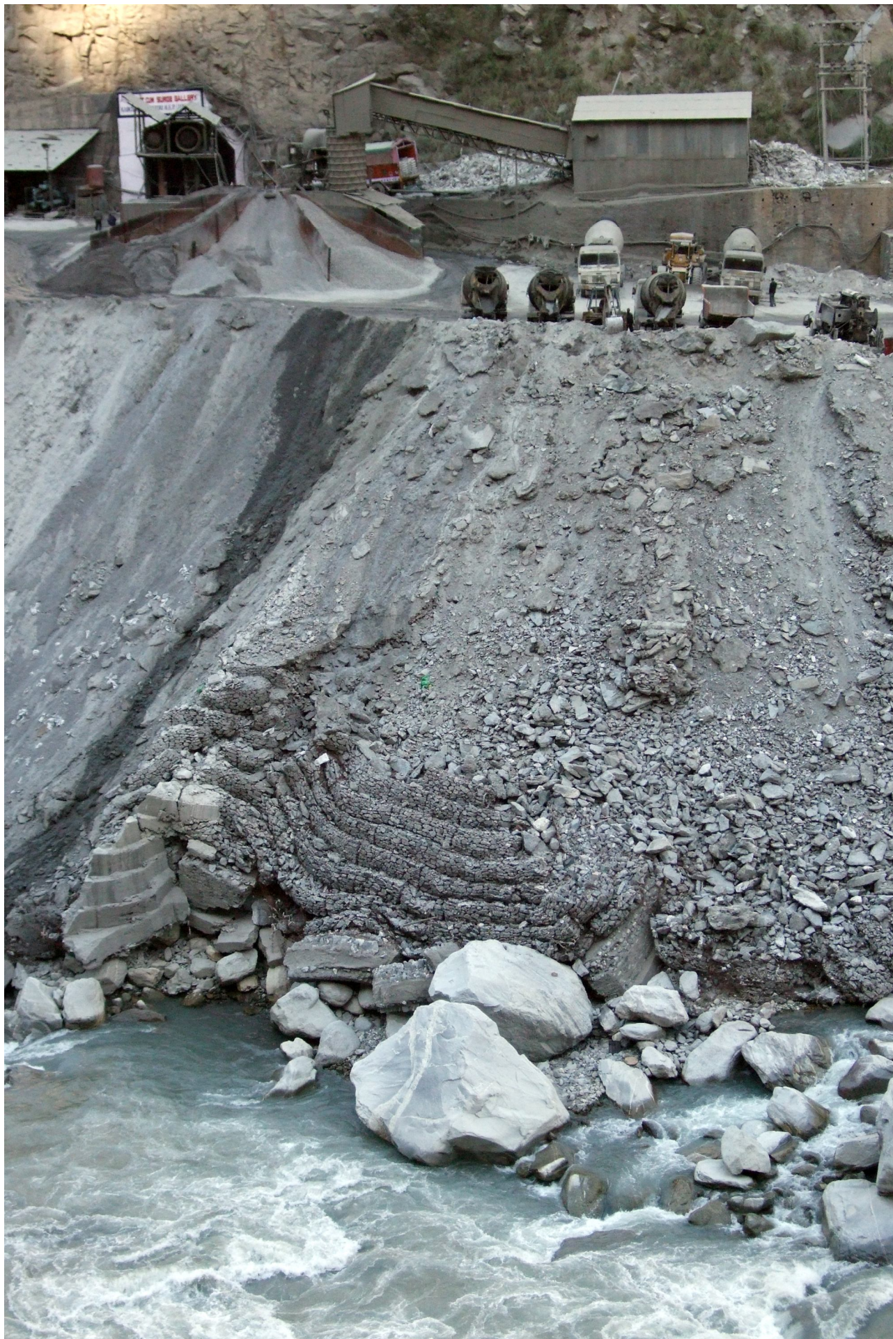
2. Photo 2 showing how the muck is flowing into the Sutlej river. Photo taken a few km downstream from the dam site on Nov 10 2010
