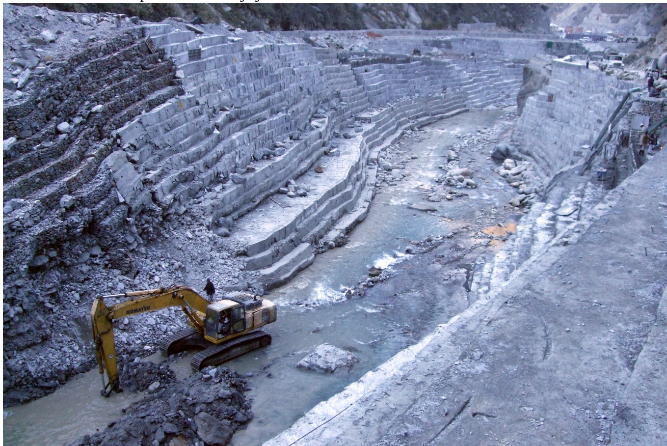
6. Photo 6 showing how the muck is flowing into the Baspa river. Photo taken about 1 km upstream from the confluence of Baspa river with Sujlej on Nov 20 2010
