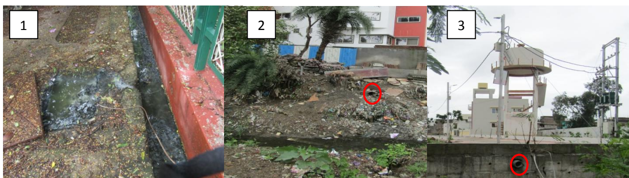
Fig. 4: Untreated Wastewater Release - 1. UDA, 2. Private Hospital, 3. Private Housing Colony
