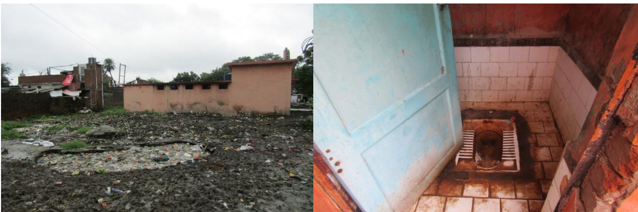
Fig. 9: Overflowing septic tank and choked toilet of Sulabh Shouchalaya in Hira Mill Ki Chawl
