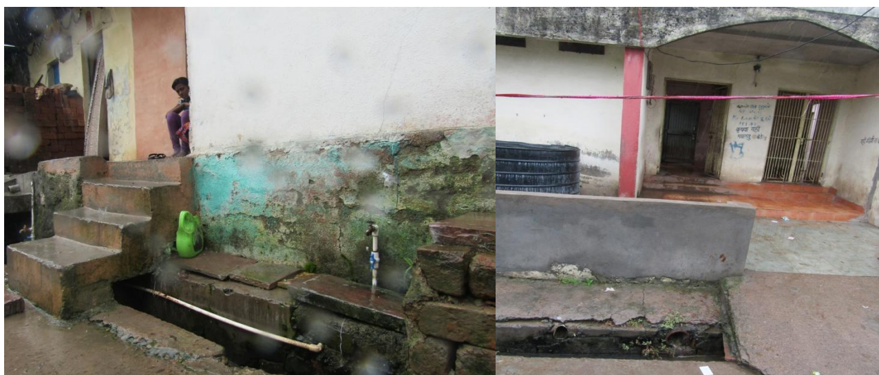
Sulabh Shouchalay community toilet as shown below.
