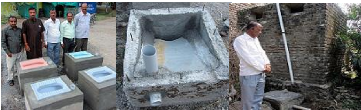
Fig. 10: The Gram Kranti Eco-bio Toilet which requires little space and the outflow is safe
