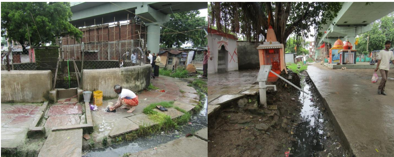
Fig. 8: Open Drain contaminating the water of the open wells and handpumps in Hira Mill Ki Chawl
