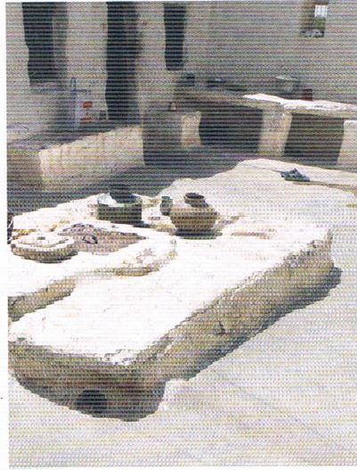
The monsoon rains are collected from the roof and the courtyard of the village houses of the desert, and stored in tanks below ground (Fig. 9 and 10).
