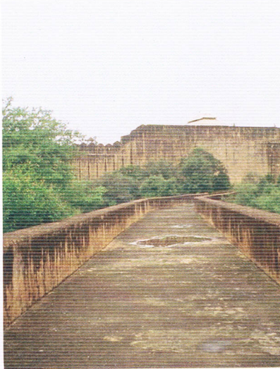
Monsoon rainwater is collected from the surrounding hills and flows through canals down into the main tank in Jaipur (Fig. 12 and 13).
