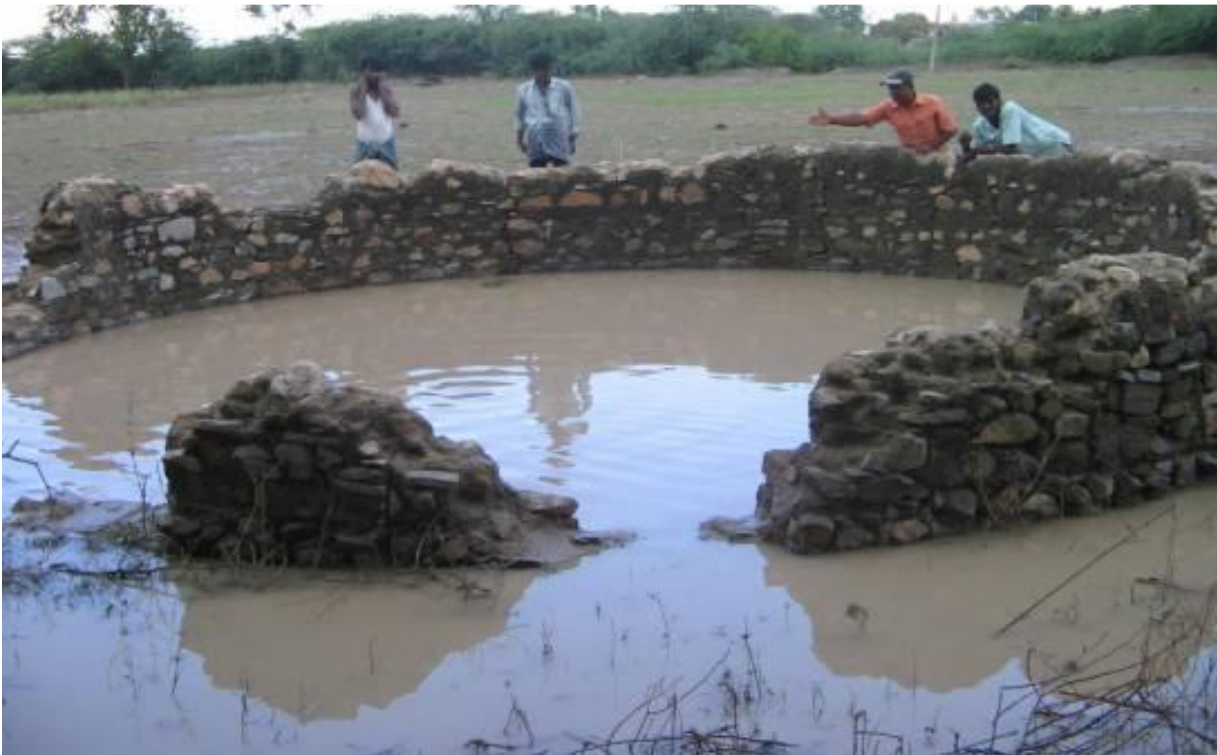
After intervention water from the well bottom was flowing like a fountain several inches thick that filled this dry well in 10 minutes
