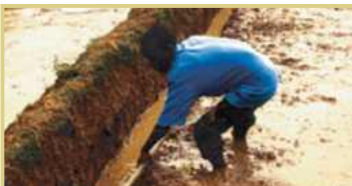
Photo 5.5 Drainage channel at the periphery
