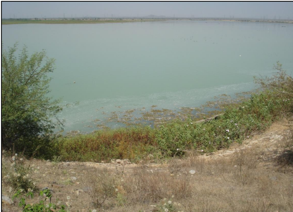
Photo 3: Ash Pond of 2340 MW Chandrapur Super Thermal Power Station (Mahagenco)
