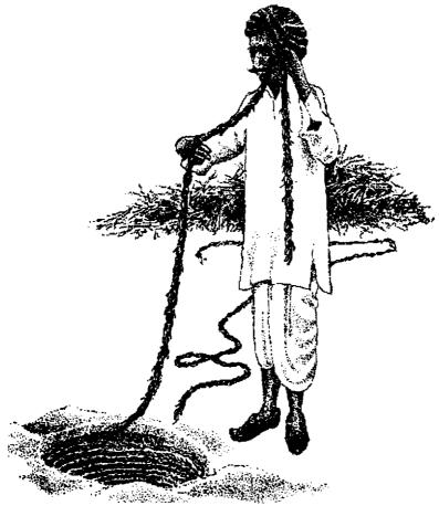
The next day more digging (the length of a few hands) takes place; a few more hands of earth is dug out and the *kundali* (coils) of rope which was fixed the previous day is then shifted to the newly dug area. The upper part of the free wall is then covered with new rope. To maintain the coils of rope on the wall, in between they are covered with *chinai* (masonry work).
