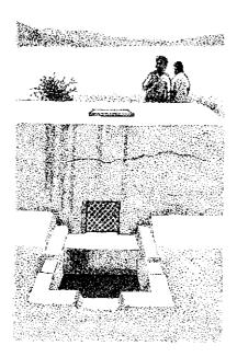
The *angan* from where rainwater is collected for the *kundi* is called *agor*. The name *agor* comes from the verb *agorna* meaning collecting. Throughout the year the *agor* is kept spotlessly clean. In fact before the rains, it is meticulously cleaned. One cannot enter the *agor* (impluvium) wearing any kind of footwear.
