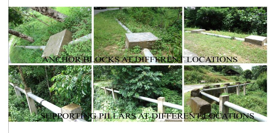
Due to the steep nature of topography, anchor blocks and RCC supporting pillars are necessary to maintain proper alignment of pipelines in w/s schemes which require high cost of projects as different from plain areas of mainland India. Often no other pipe alignment options are available except to go through difficult terrain/alignment often crossing landslide prone areas as in the case of w/s project for Dimapur Town.
