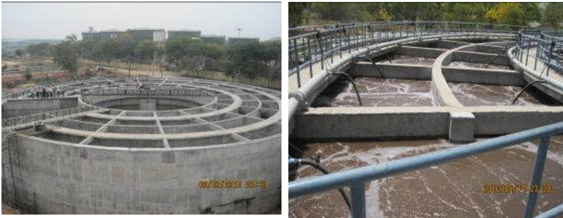
Figure 5.15 Left is the bioreactor during construction; Right is the bioreactor after commissioning showing the rich MLSS culture in the annular plug flow reactor
