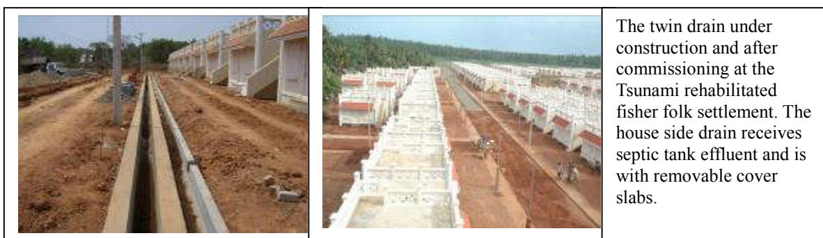
Figure 3.11 Twin drain system
