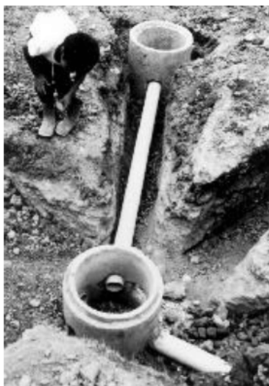
Figure 8.6 Junction chamber for simplified sewerage using larger diameter concrete pipes, used in Guatemala
