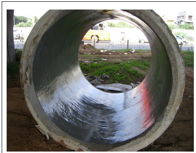
Figure 3.58 RCC Sewer pipe with protective coating
