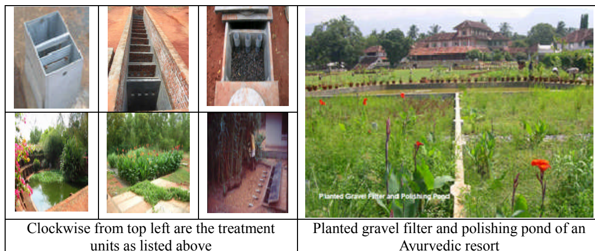
Figure 8.14 Typical DEWATS treatment plant components
