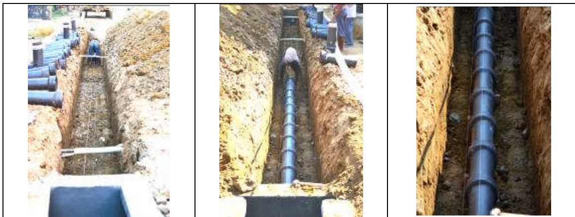
Figure 3.50 A simpler approach to initial laying and aligning the SW sewers by the two tight twines one on crown and one on mid diameter are used
