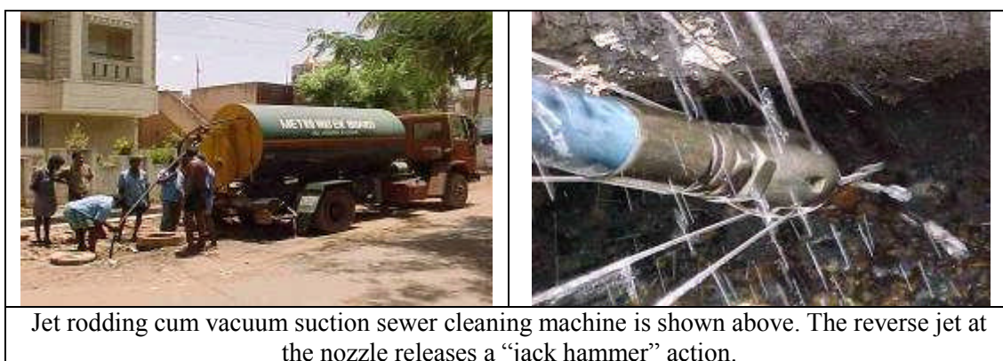
Figure 3.10 Jet rodding cum vacuum, suction sewer cleaning machine
