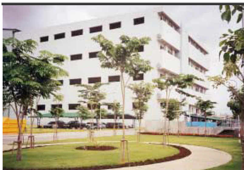
Figure 5.71 Yannawa STP, Thailand
