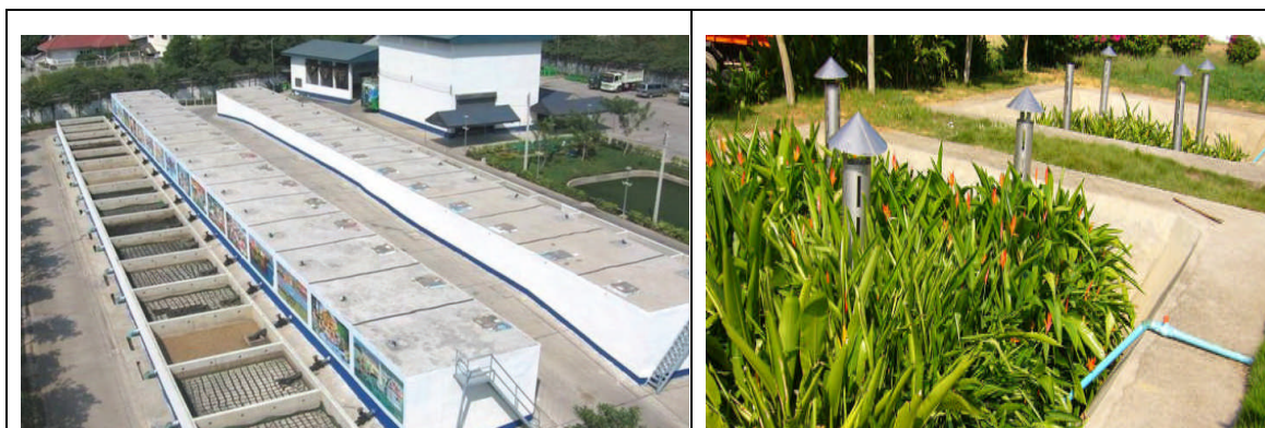
The Nonthaburi Municipality’s septage treatment facility has 30 anaerobic digestion tanks and is one of the best run facilities of its kind in Thailand. As part of a pilot project to improve septage treatment in Lampang, the Asian Institute of Technology partnered with Lampang Municipality to build a treatment facility that uses a grid of reed beds to treat septage leachate to secondary levels.
