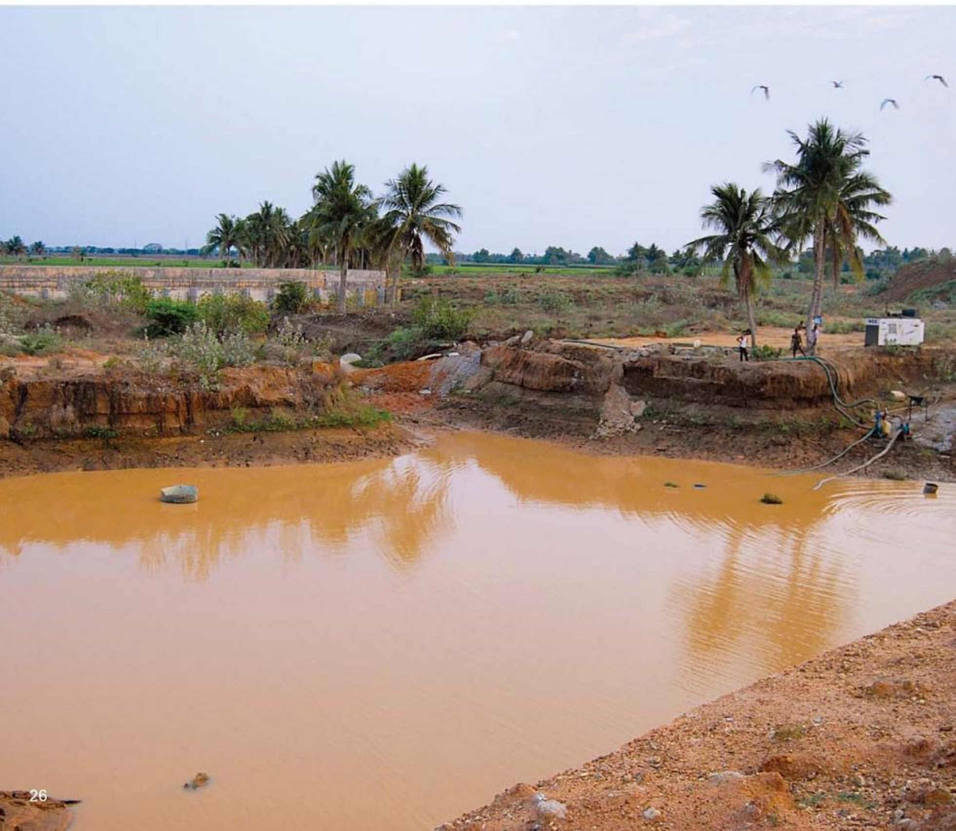
Artificially excavated pond at Polavaram Project site
