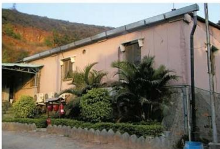
Rooftop Rainwater Harvesting at Vizag Project site
