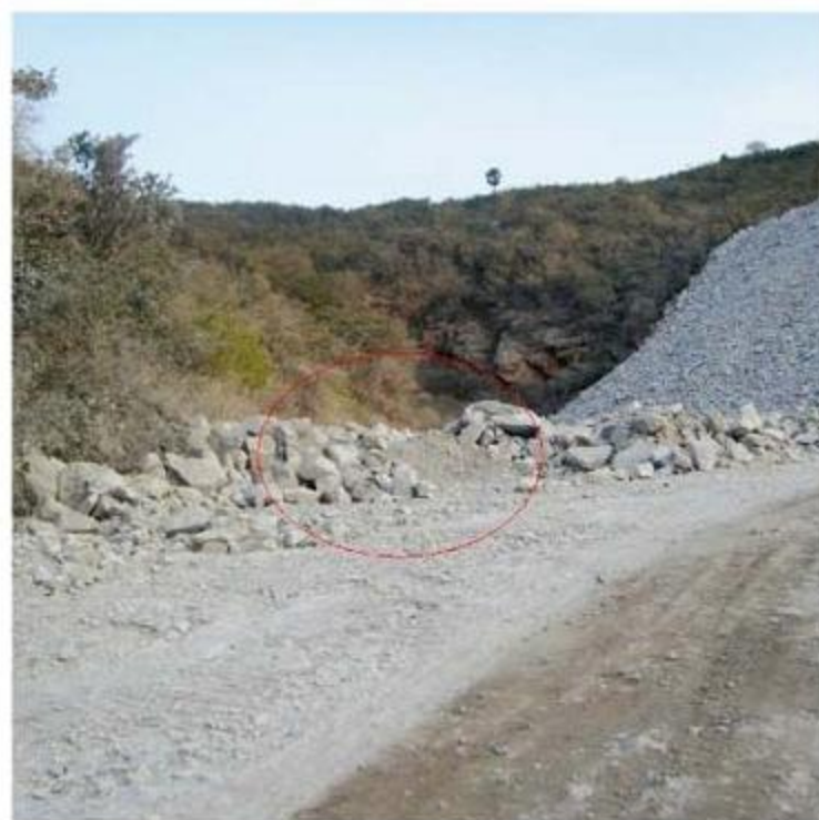
Embankment created near natural pond at Vizag Project site
