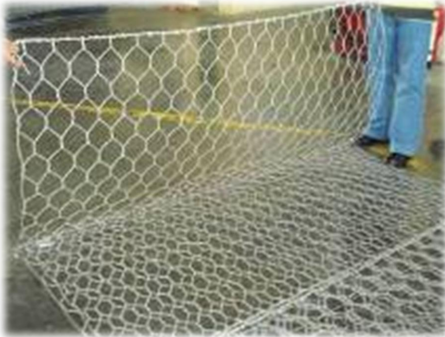
Figure 8-4: Straightening out of DT mesh panels of folded gabion unit
