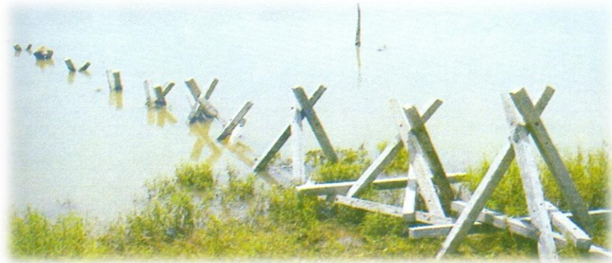
Figure 6-2: Typical RCC porcupine screen
