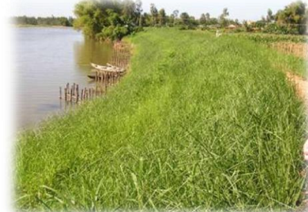
Figure 4-4: Bank after the vetiver implementation
