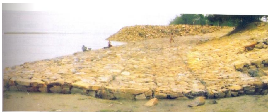
Figure 4-8: A typical bank pitching in wire crates
