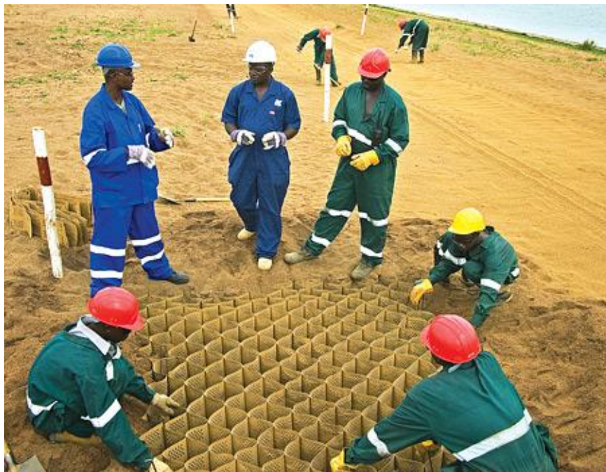
Figure 4-7: A typical geo-cell being prepared at site
