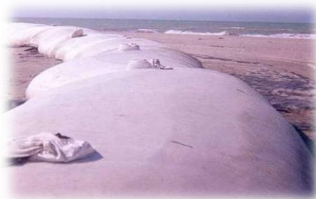
Figure 2-5: Geo-textile tube
