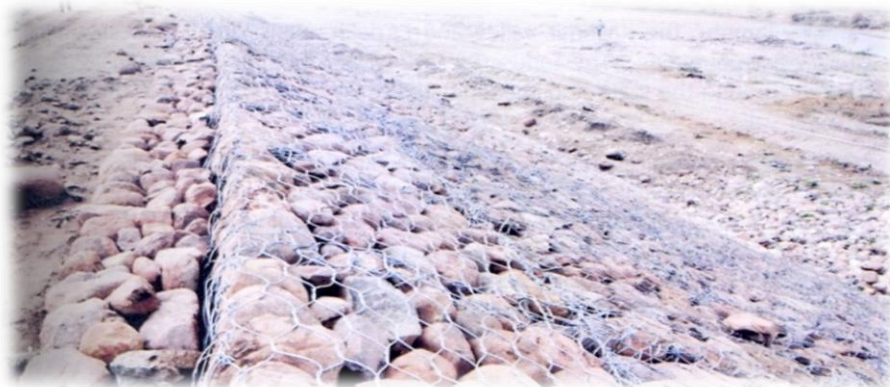
Figure 4-9: A typical bank pitching in crates
