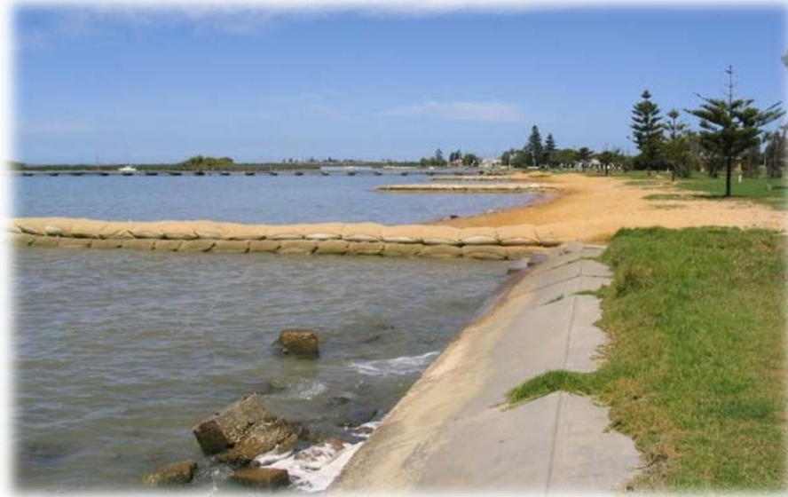
Figure 5-7: Spur along with bank protection using geo-textile
