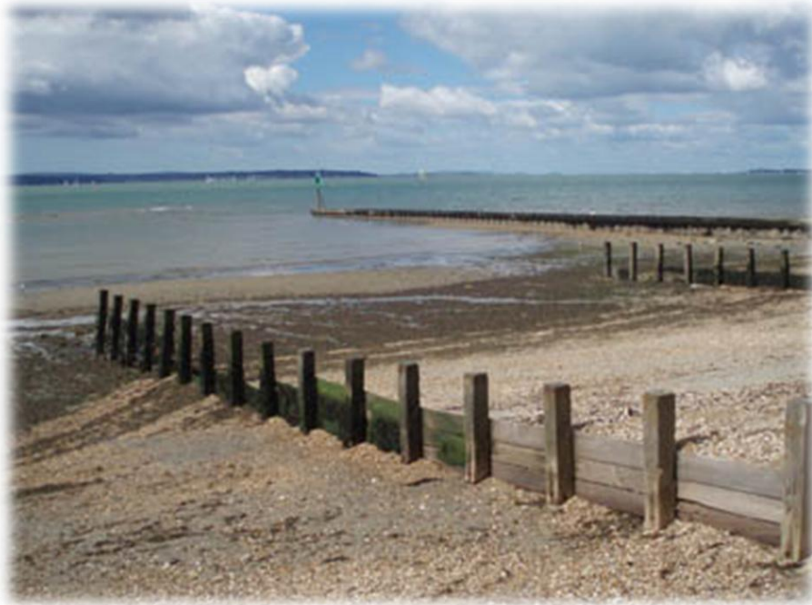
Figure 5-3: Permeable spurs constructed with timber
