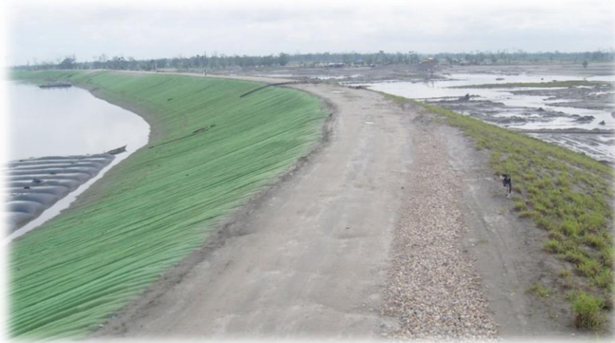
Figure 3-9: A typical completed embankment with road on crest
