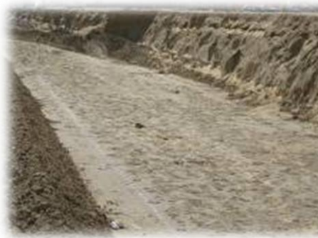
Figure 8-2: Formation of excavated surface
