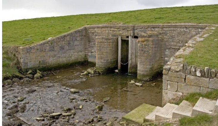
Figure 7-6: A typical gated sluice drain
