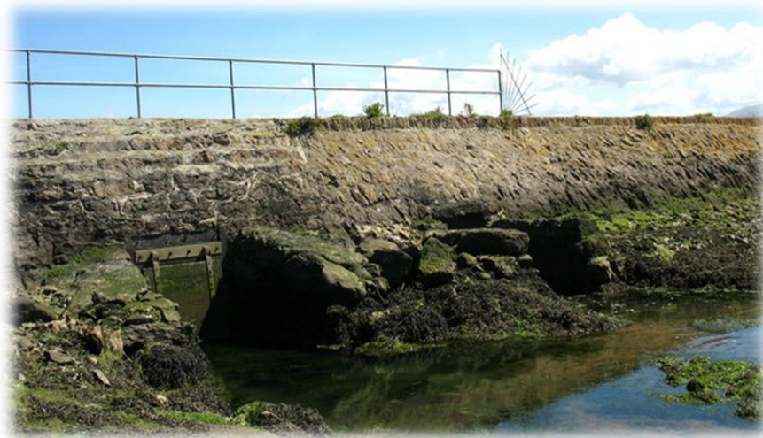
Figure 7-4: A gated sluice
