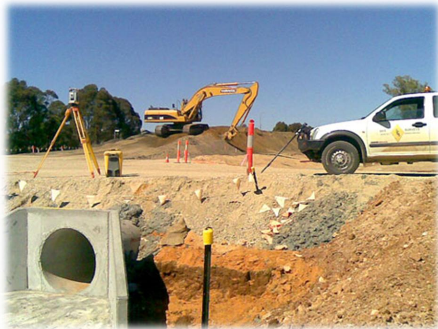
Figure 7-2: cross drain under the embankment
