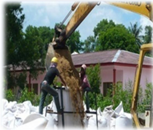
Figure 8-11: Filling of geo-bags
