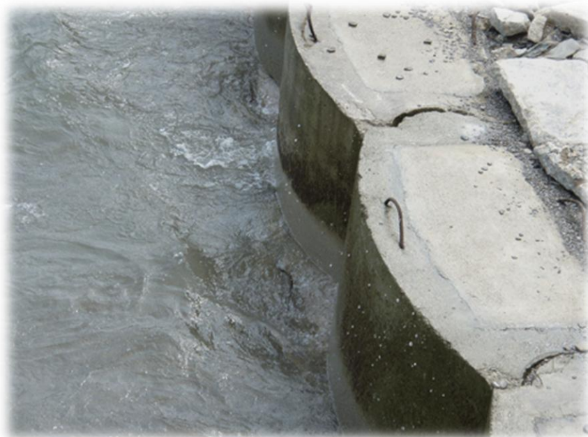
Figure 4-11: Use of cement blocks in bank protection
