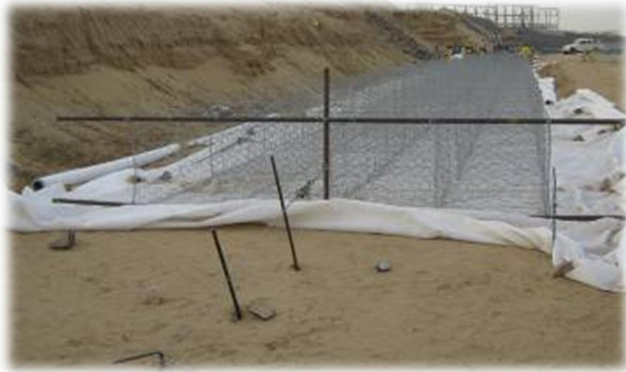
Figure 8-7: Stretching the gabions
