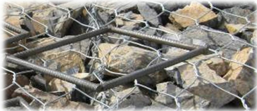
Figure 8-8: Boulders filled in gabions
