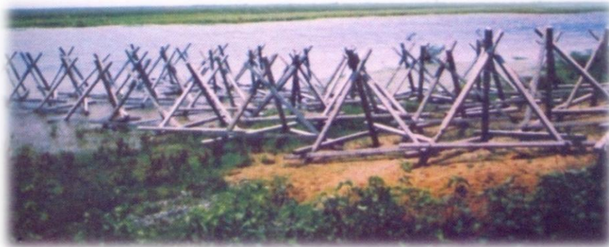
Figure 6-4: RCC porcupine spur
