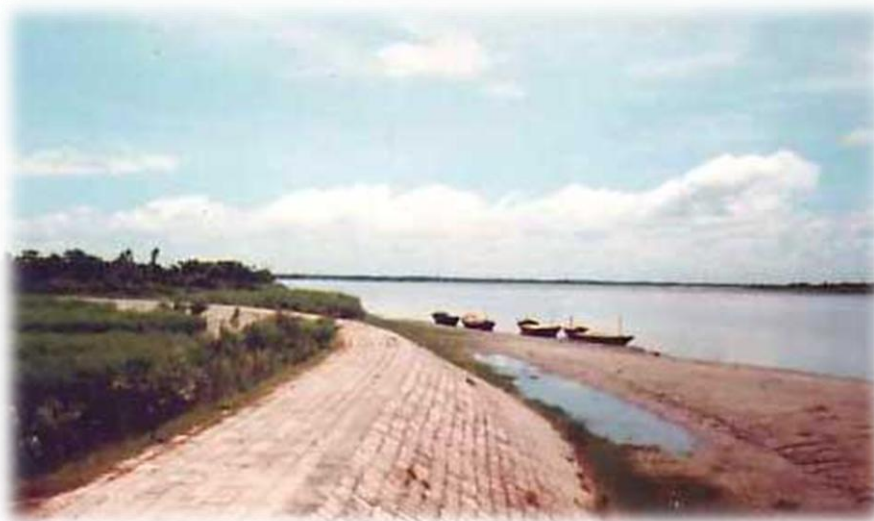
Figure 4-1: A typical bank protection work
