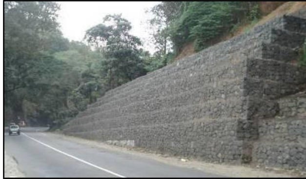
Figure 8-1: Gabion retaining wall
