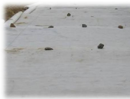
Figure 8-3: Geo-textile laid out on rolled surface
