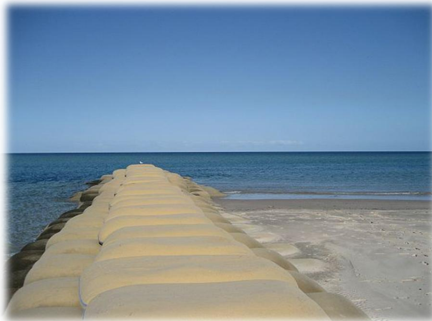
Figure 5-6: Spur using geo-bags
