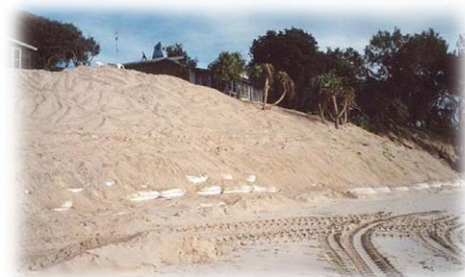
Figure 4-13: Bank after implementation of geo-bags
