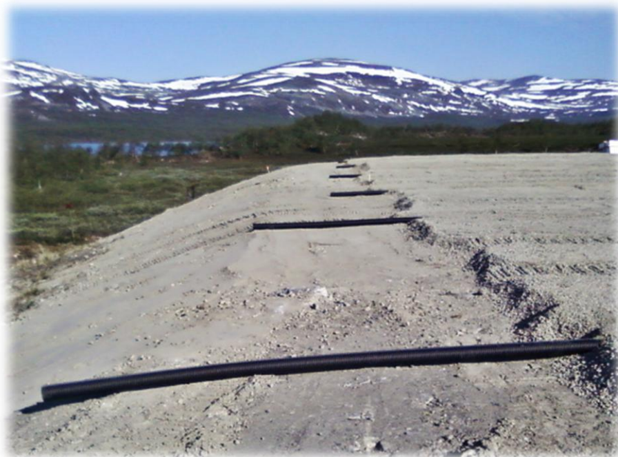
Figure 3-7: Provision of drain pipe
