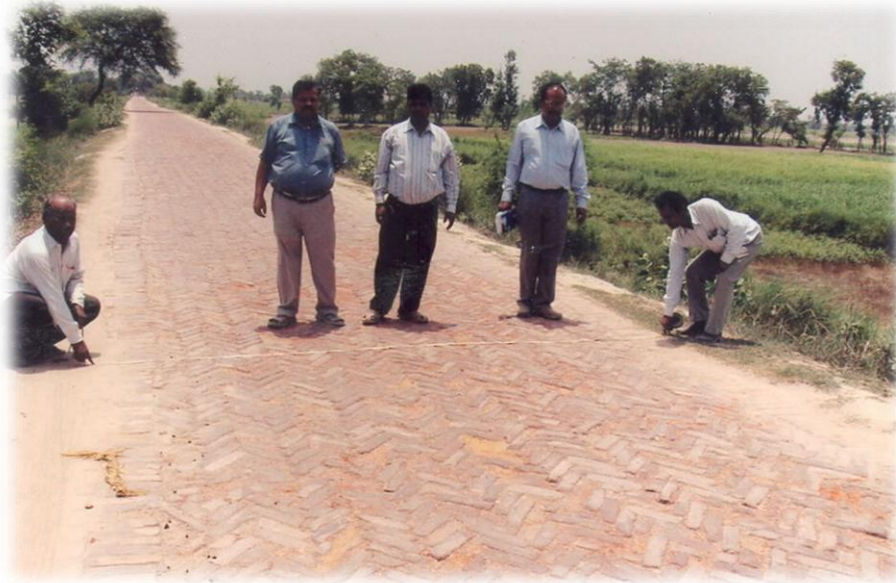
Figure 3-4: An embankment crest with brick soling
