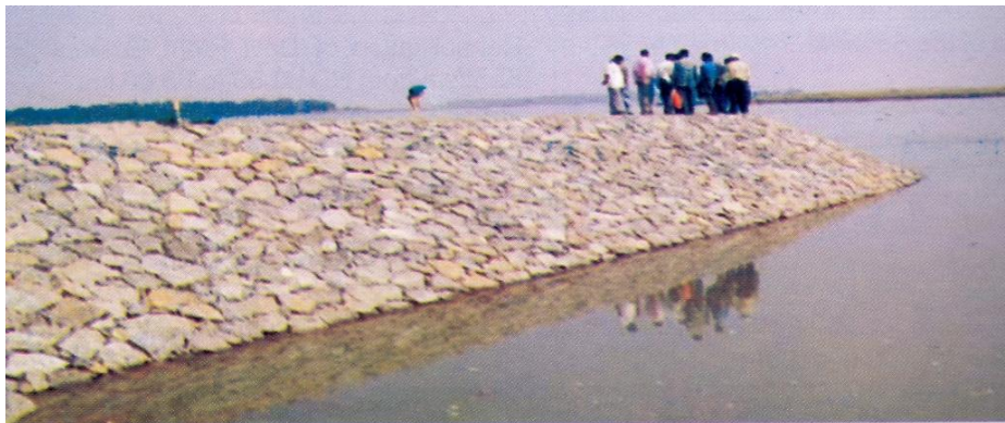
Figure 5-1: Spur built with boulders
