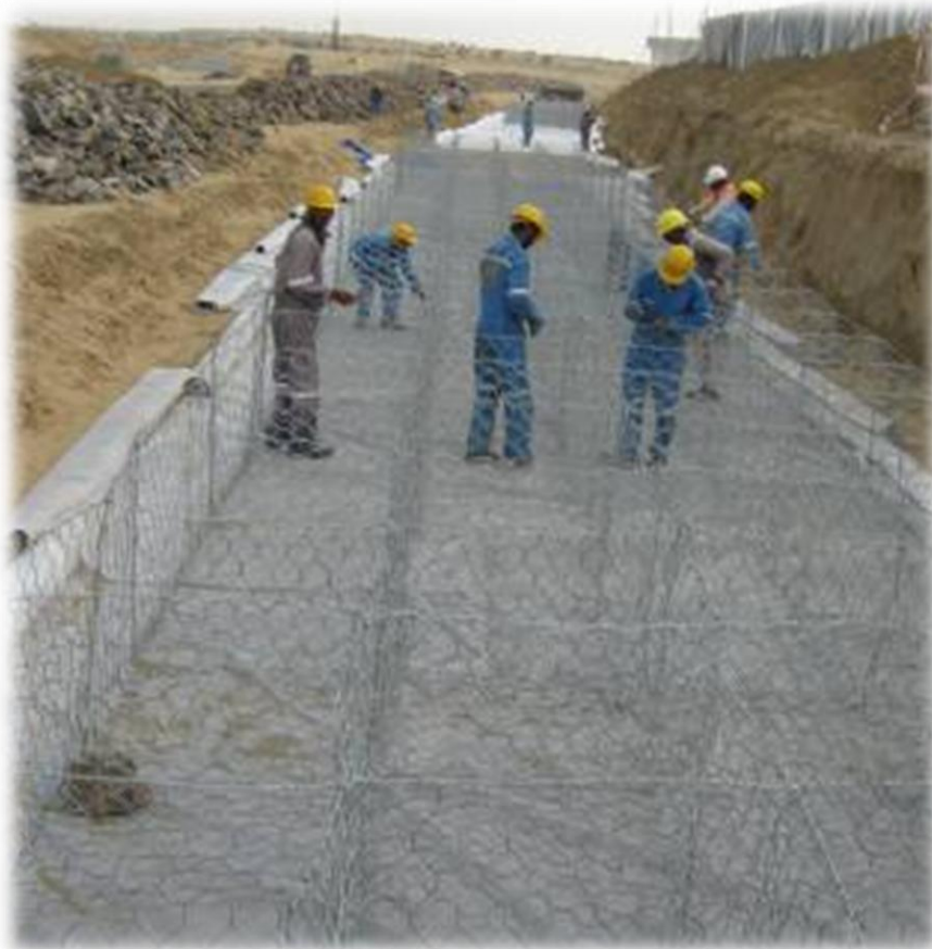
Figure 8-6: Laying and connecting all adjacent gabions
