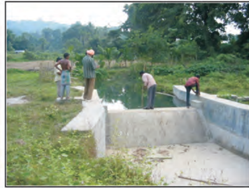
Fig 10.31 A Check Dam
