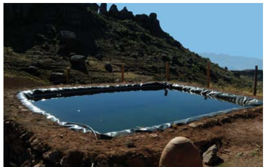
New, small reservoir, collecting water from permanent springs. (photo: Johanna Götter)
