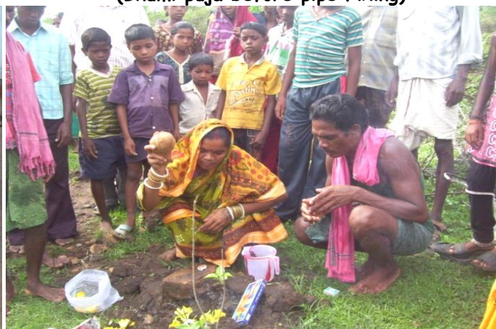
(Bhumi puja before pipe Fixing)
