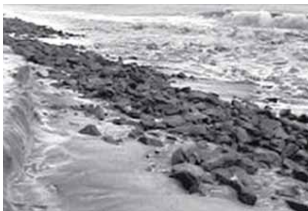
Figure 8 : Coastal hazard impact
