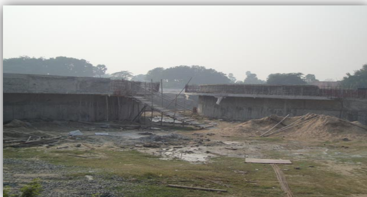
Figure 6-5: Surface water supply scheme under construction
