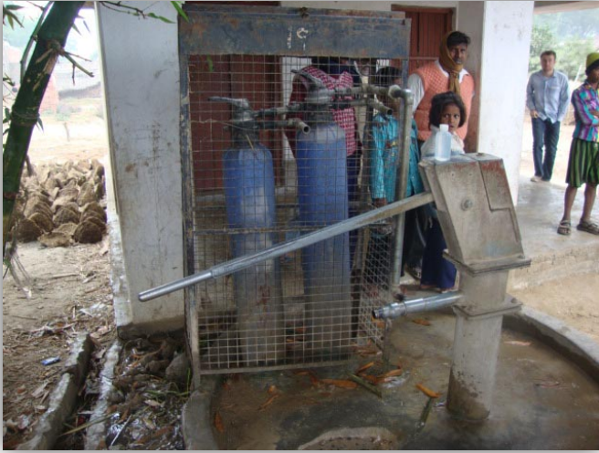
Figure 6-9: Well head adsorption filter
