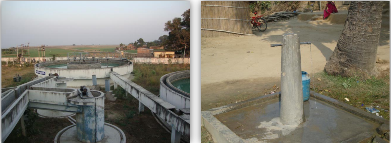
Figure 6-1: Mozempur water supply plant (left) and distribution (right)
