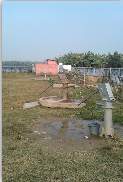
Figure 6-10: Three hand pumps without filter
