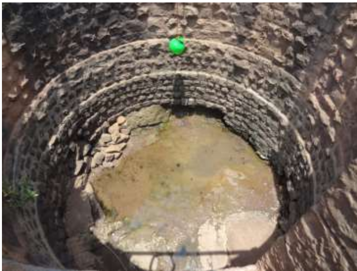
Image 50 Water level in drinking water well during mid summer
