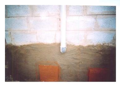
Avoiding detachable slabs behind the chamber but constructing with a hole and closing the hole with bricks and Mud Mortar can reduced the RCC cost.
