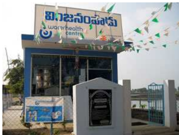
The WHI plant in Vinjinampadu
