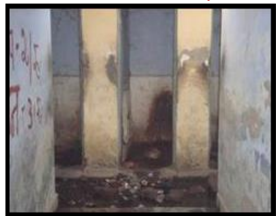
Bad Condition of Community Toilets
