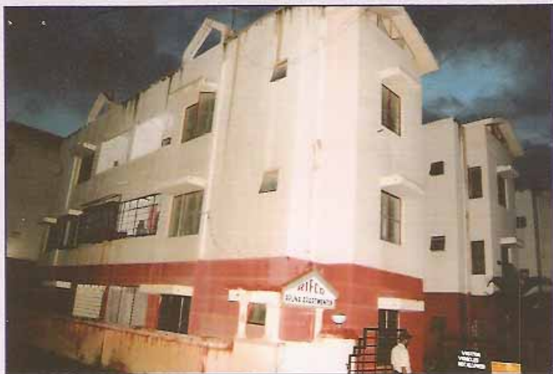
RIFCO Housing complex constructed on Konena Agrahara Tank Bed
