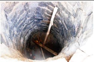
'Septic Tank', constructed like a pit latrine
