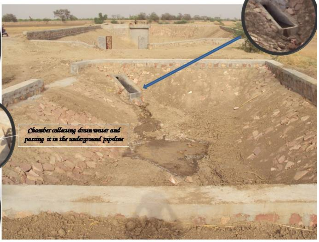
Underground drain connection (connecting drain inside the School Pond with that of the Cattle Pond)
