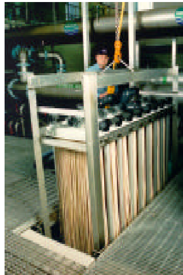
Installation of a ZeeWeed membrane in the process tank
