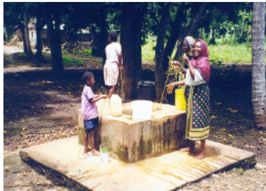
The classical dug well with all the conditions conducive to contamination
