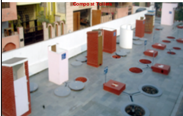
Panoramic View of Different Designs of Sulabh Two-Pit, Pour-Flush, Compost Toilets
