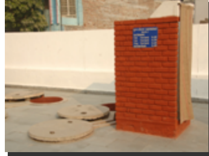
Cost – US $152 (Rs. 7600) Brick wall with jute curtain.
