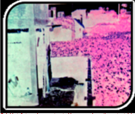
The Sulabh toilet can be constructed in areas where the water-table is high, in waterlogged, flood prone and high sub-soil water areas where the pits could be raised.
