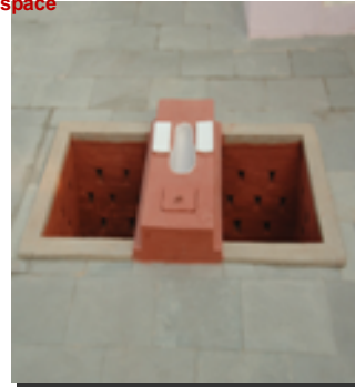
Sulabh pour-flush toilet for least space with the toilet on top of the pits
