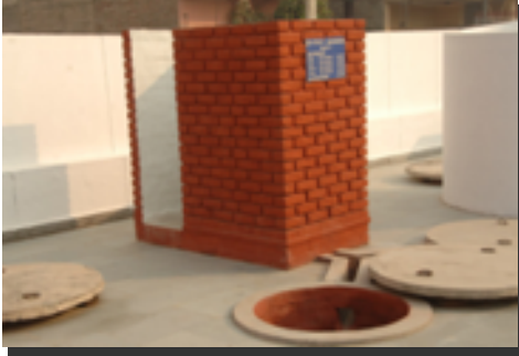
Cost – US $145 (Rs. 7250) Brick wall with no door.
