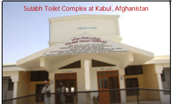
Sulabh Toilet Complex at Kabul, Afghanistan Even when the temperature in Kabul went down to -30 C in 2007, these biogas plants worked very well. Hence this technology is suitable for both cold as well as warm climates
