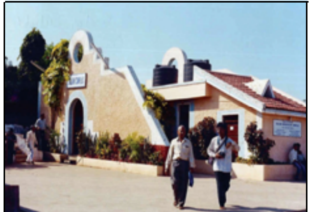
Sulabh Toilet Complex at Donapaula, Panji, Goa.
