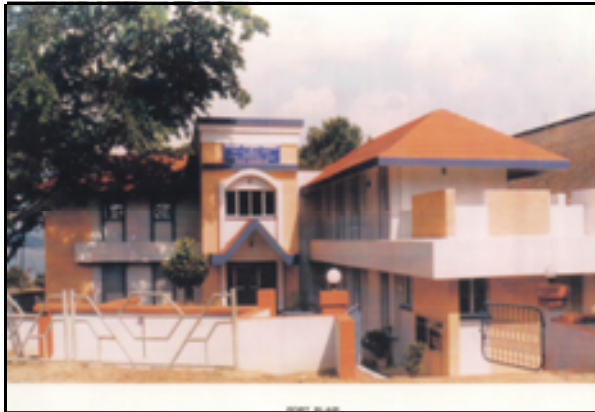
Sulabh Toilet Complex with Night Shelter, Port Blair, Andaman and Nicobar
