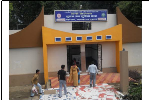
Sulabh Toilet Complex at Vishwakarma Nagar, Bhopal, Madhya Pradesh
