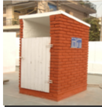
Cost – US $185 (Rs. 9250) Toilet walls made of bricks with roof and wooden door- more expensive.
