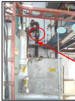
Return Line Of Chilled Water
