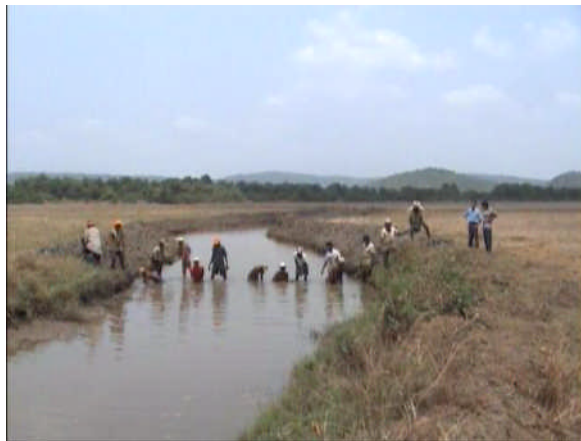
De-Silting of Nallah.
