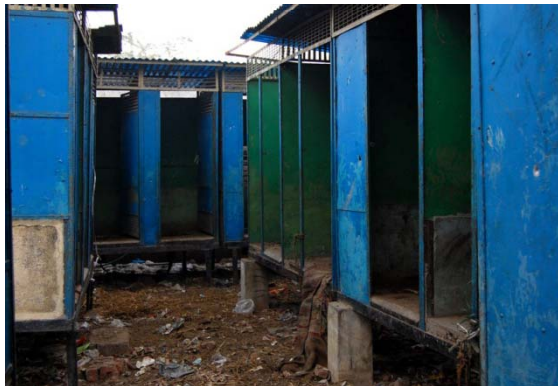
Community Toilet complex in Delhi
