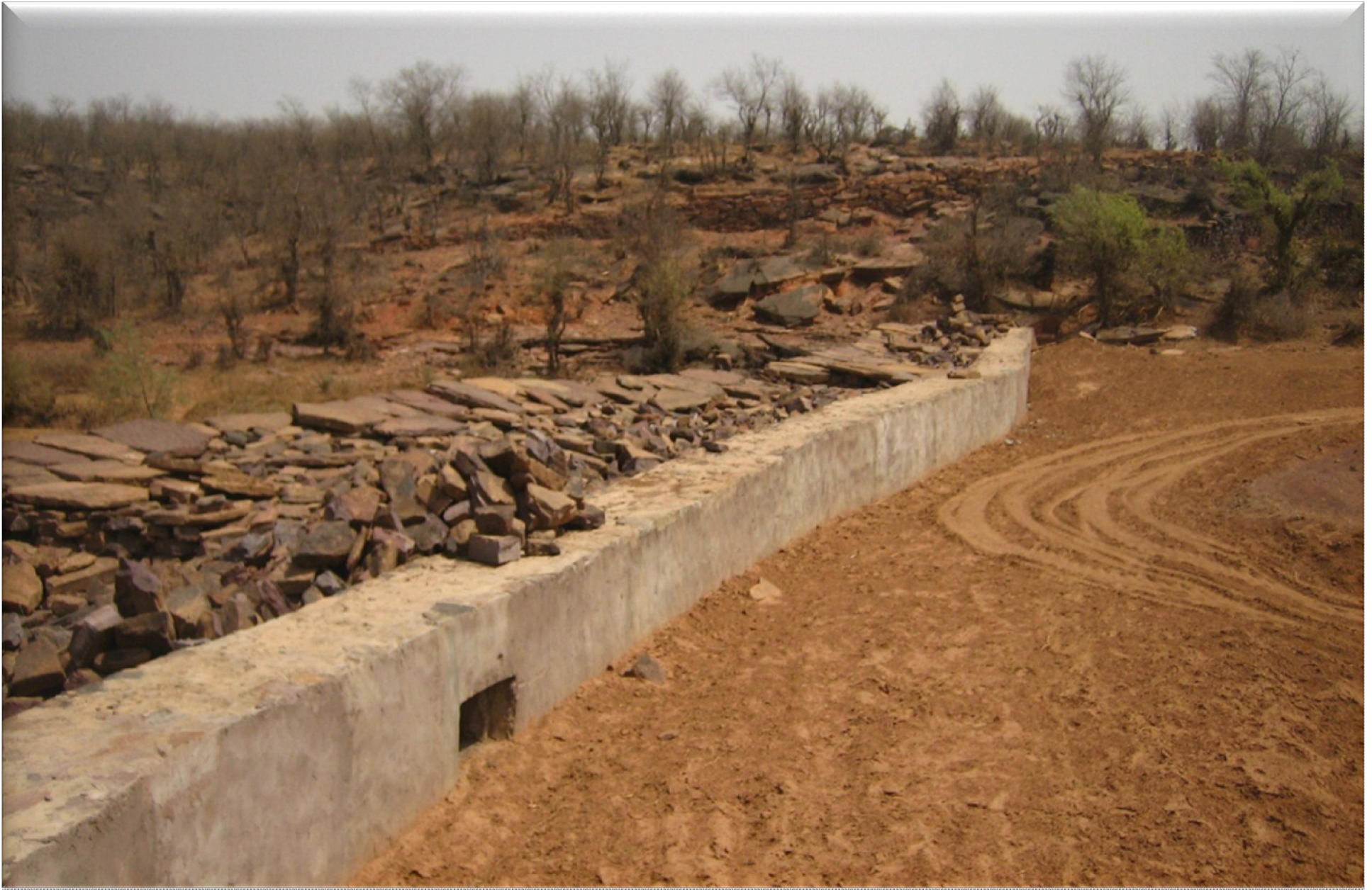
A Rainwater harvesting structure : MEDHBANDHI
