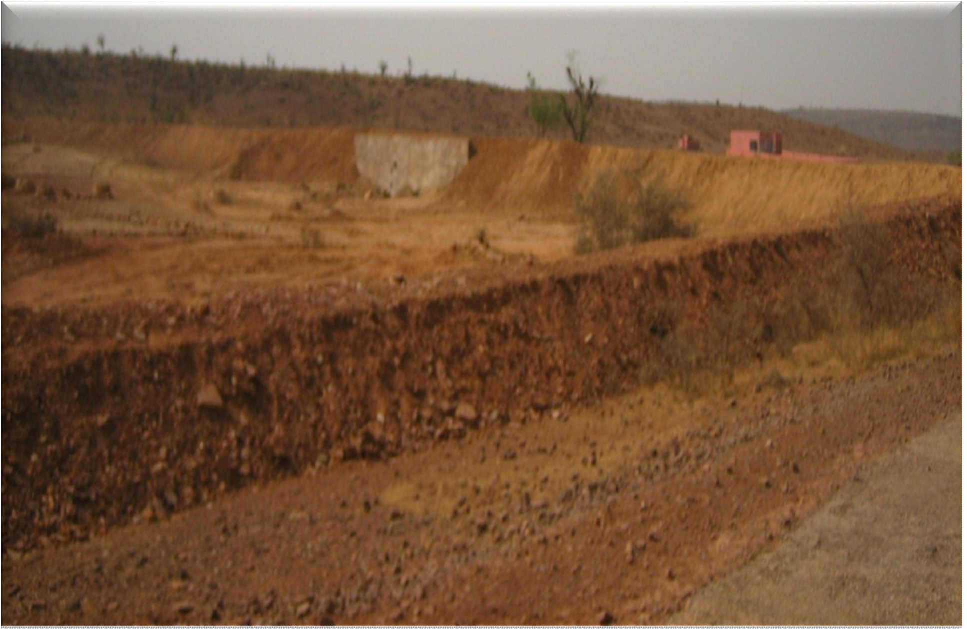
A Rainwater harvesting structure : BANDH
