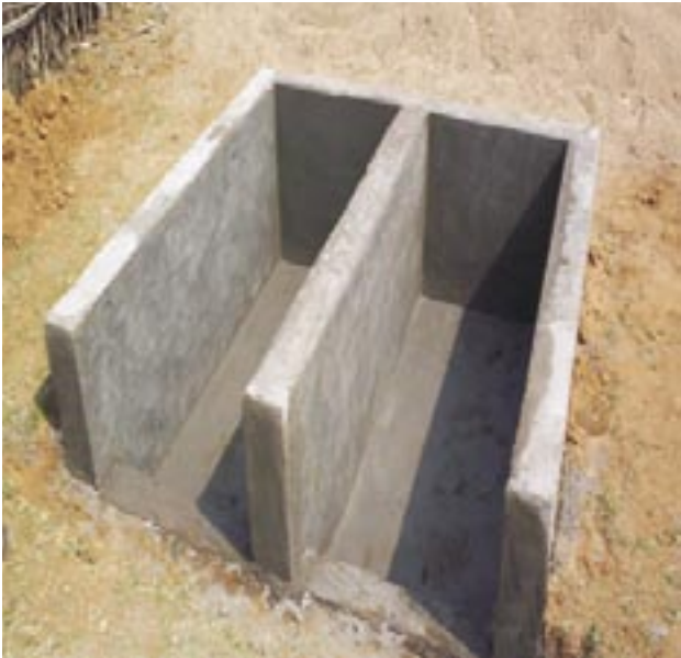
Construction of eco-san base
