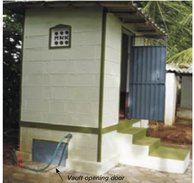
Eco-san Toilet - Vault opening door
