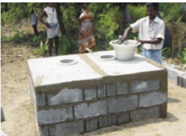
Construction of eco-san platform
