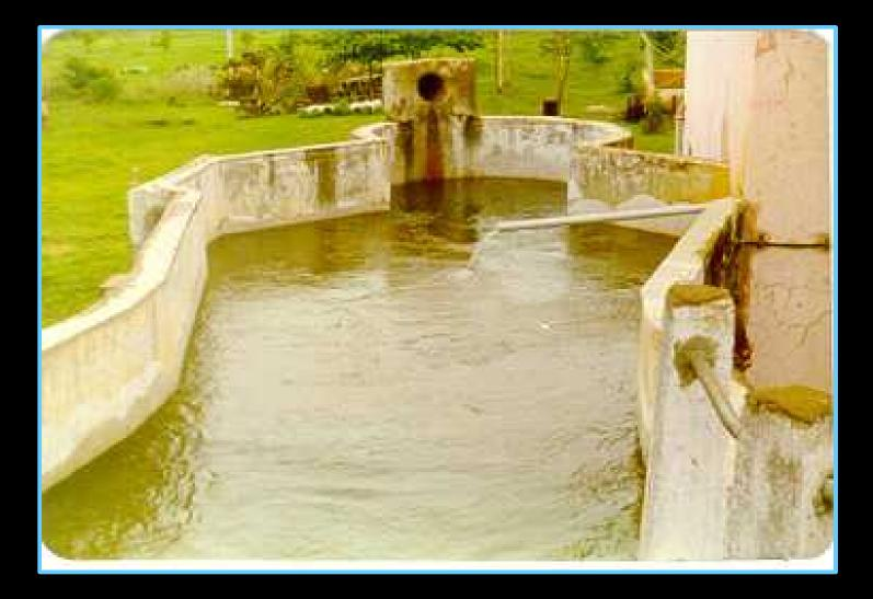
Single point addition of coagulants - Not conducive to effective mixing
