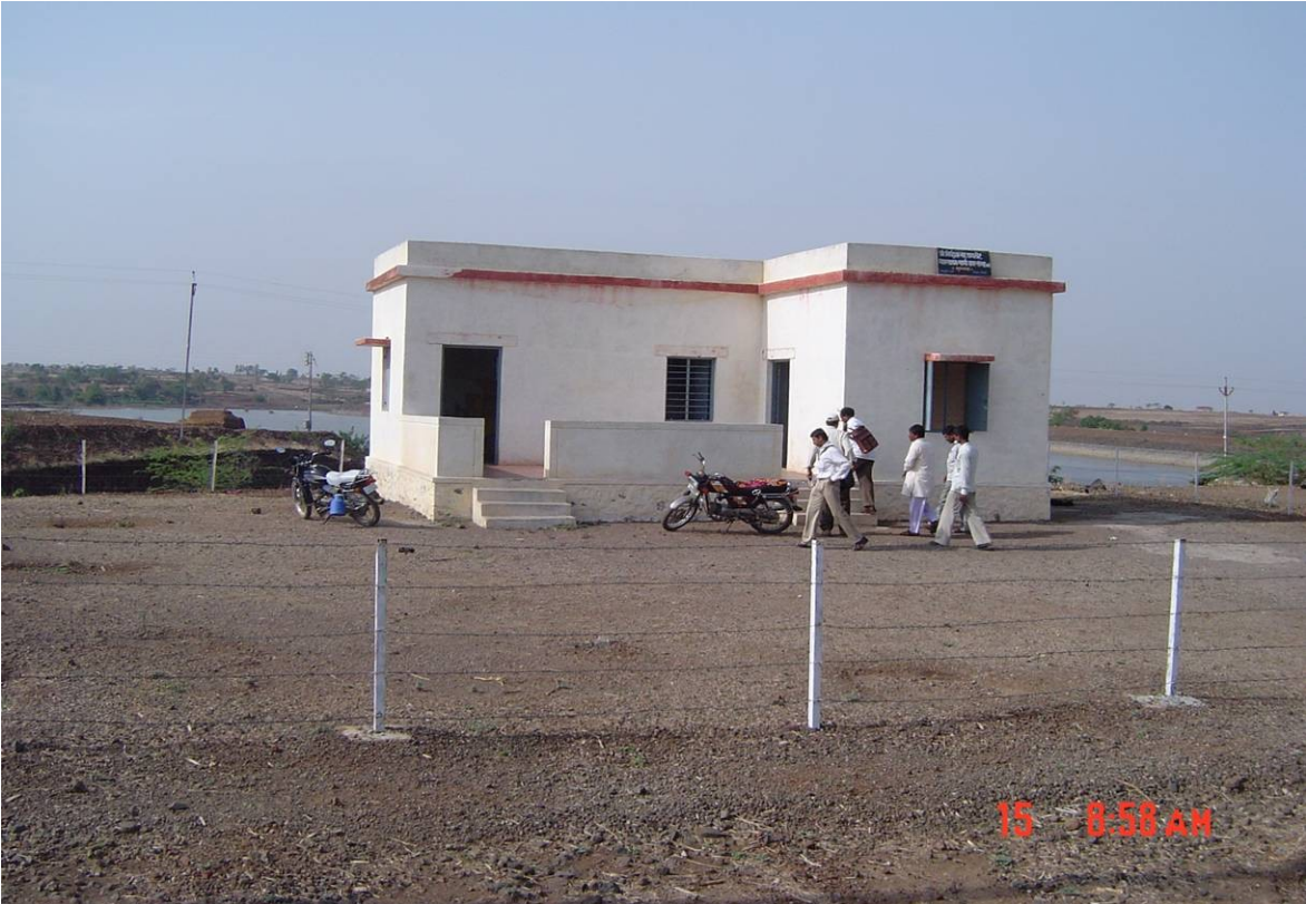
WUA Office on the Background of Storage Tank at Gugwad, Dist : Sangli
