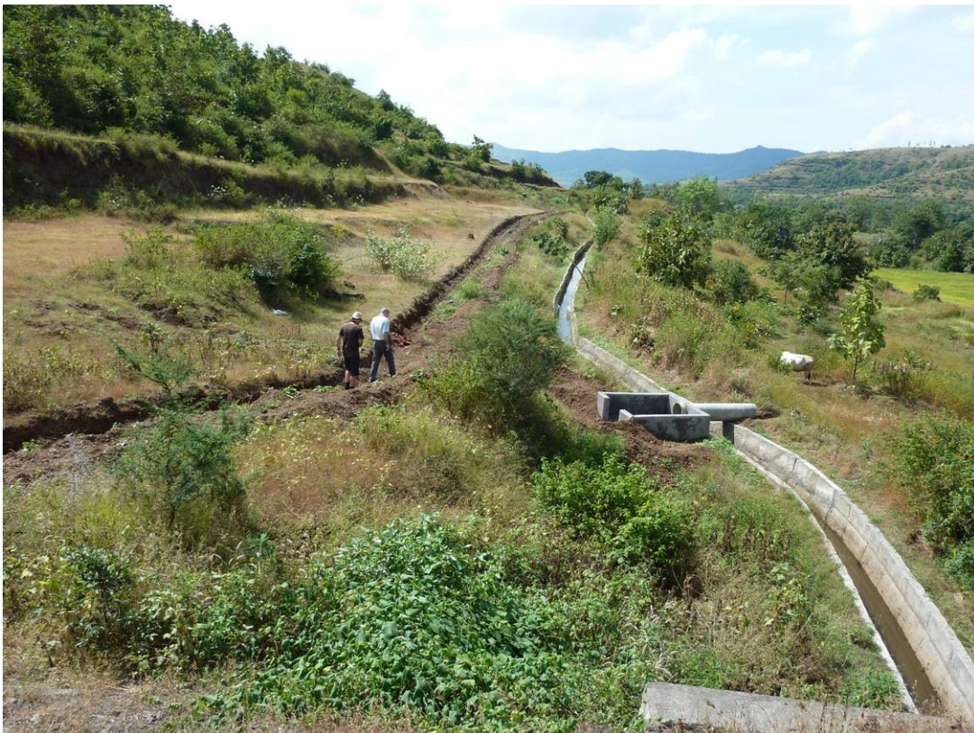
Varve Tank : Lined Canal (120 l/s) with catch water drain.
