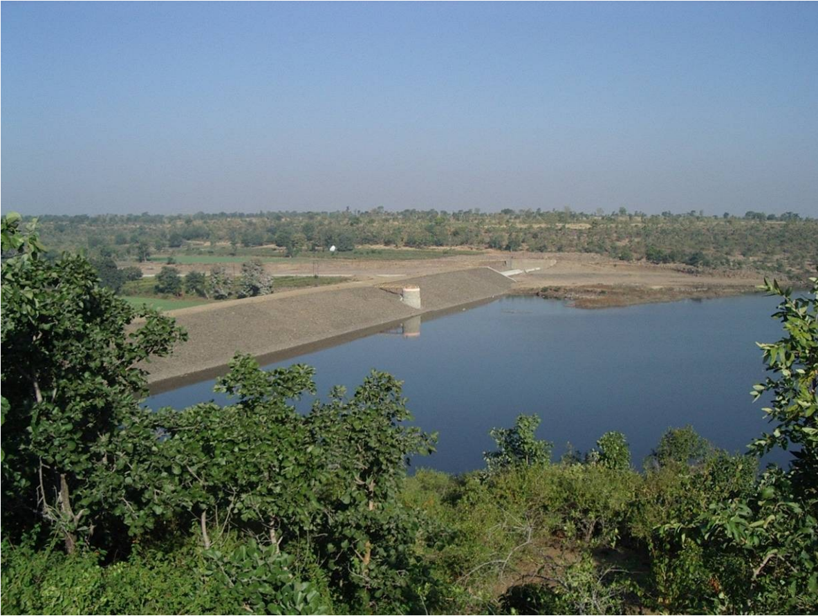
Storage Tank at Kasari, Taluka- Lonar, District- Buldhana
