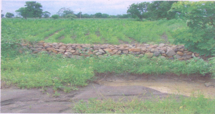
Soil deposited near a boulder waste weir
