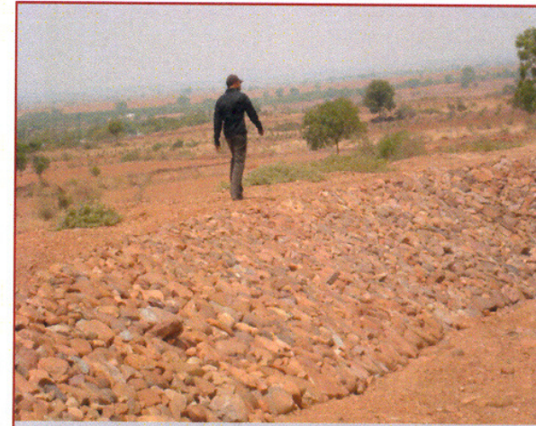
A well constructed Stonebunding in Teliki – 2/5/2009
