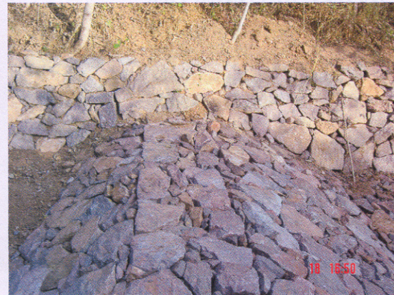
Top-view of Rock-fill Dam
