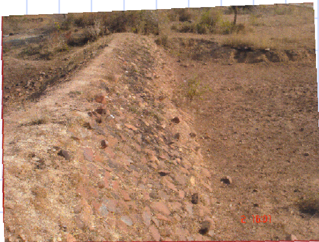
A well constructed earthen dam in Badiselvanka village under CBP – Date: 1/4/2009
