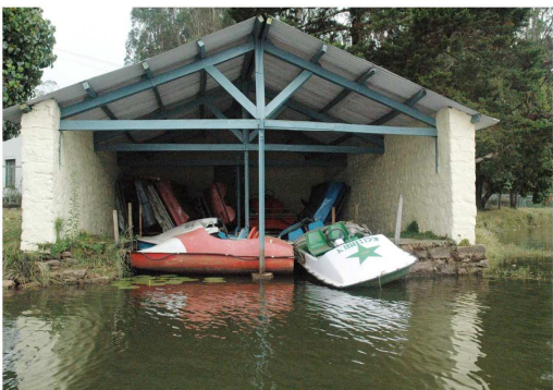
Damaged fiber glass boats
