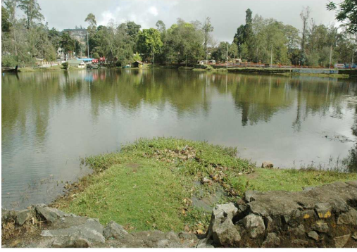
Siltation inside the Lake area
