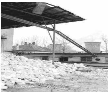
Figure 23.3. Storage of solids
