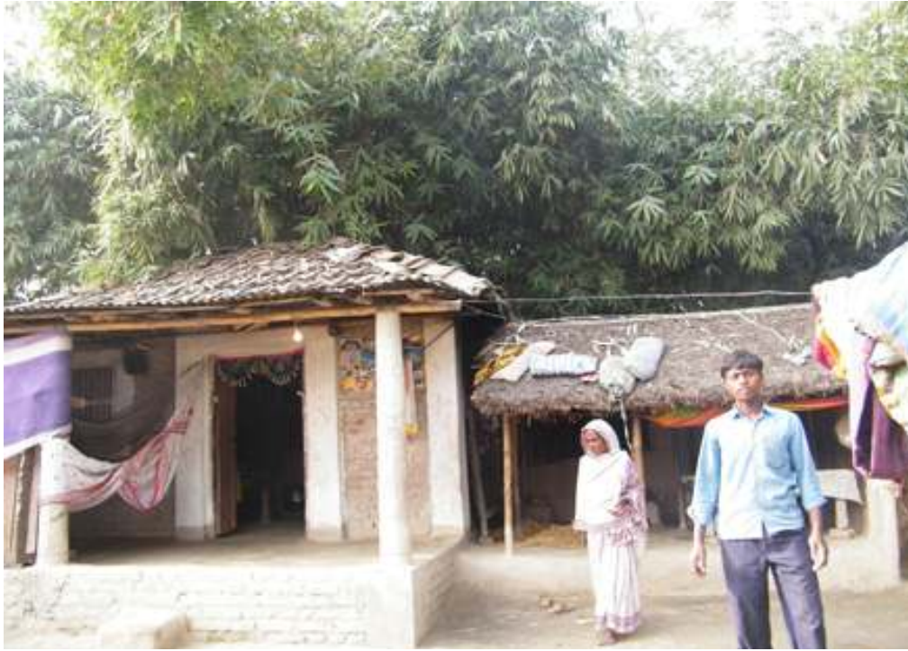
Fig 3.10 An Indira Awas Yojana house of brick and cement, tile with bamboo roof, cement columns and mud-thatch-bamboo sleeping quarters as additional room.
