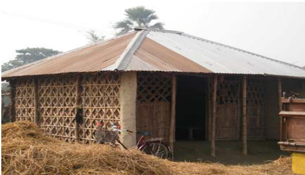
Fig 3.9 A 'fusion' house built by an affected family themselves. Gi-sheet roof, bamboo jaali and bamboo slats walls, cement 'columns', bamboo pillars, bamboo roof structure
