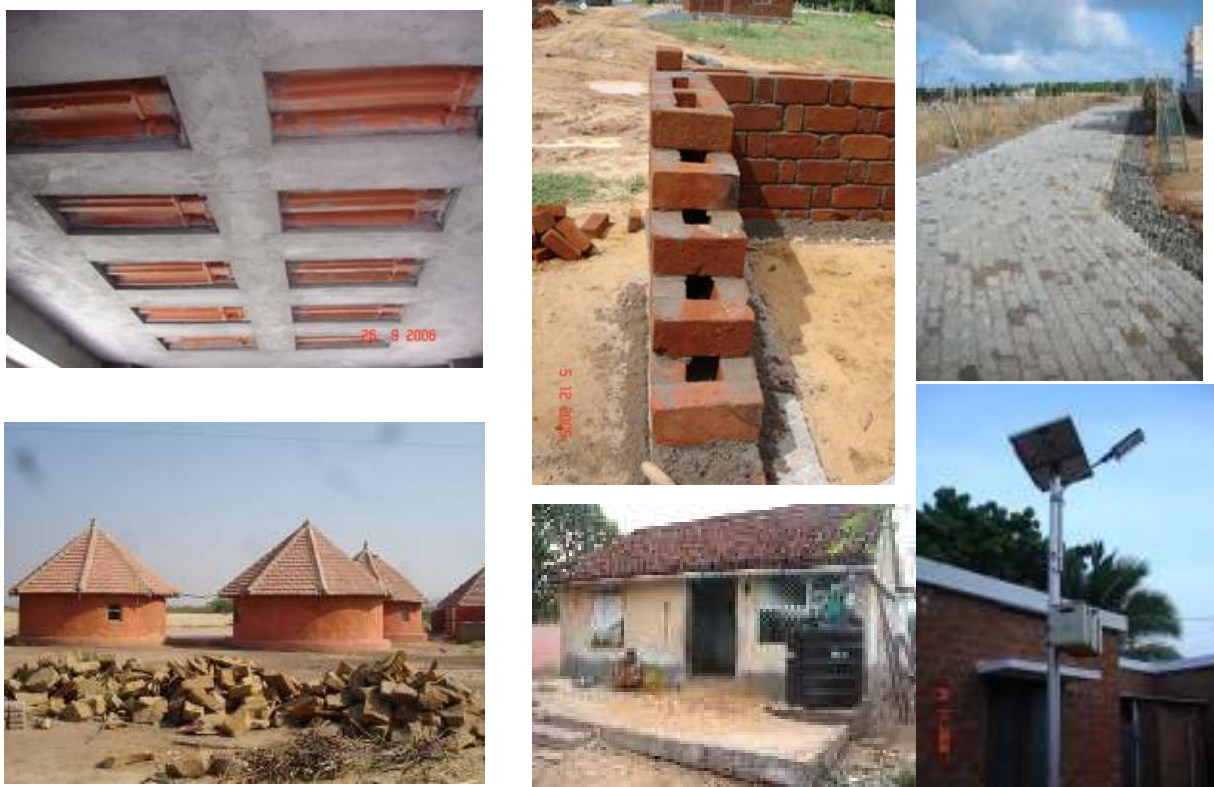
Fig 3.8 Filler-slab roof, rat-trap bond walling, permeable roads and drains (water management), ‘pucca’ brick and tile bhungas, rain-water harvesting, solar street lights.
