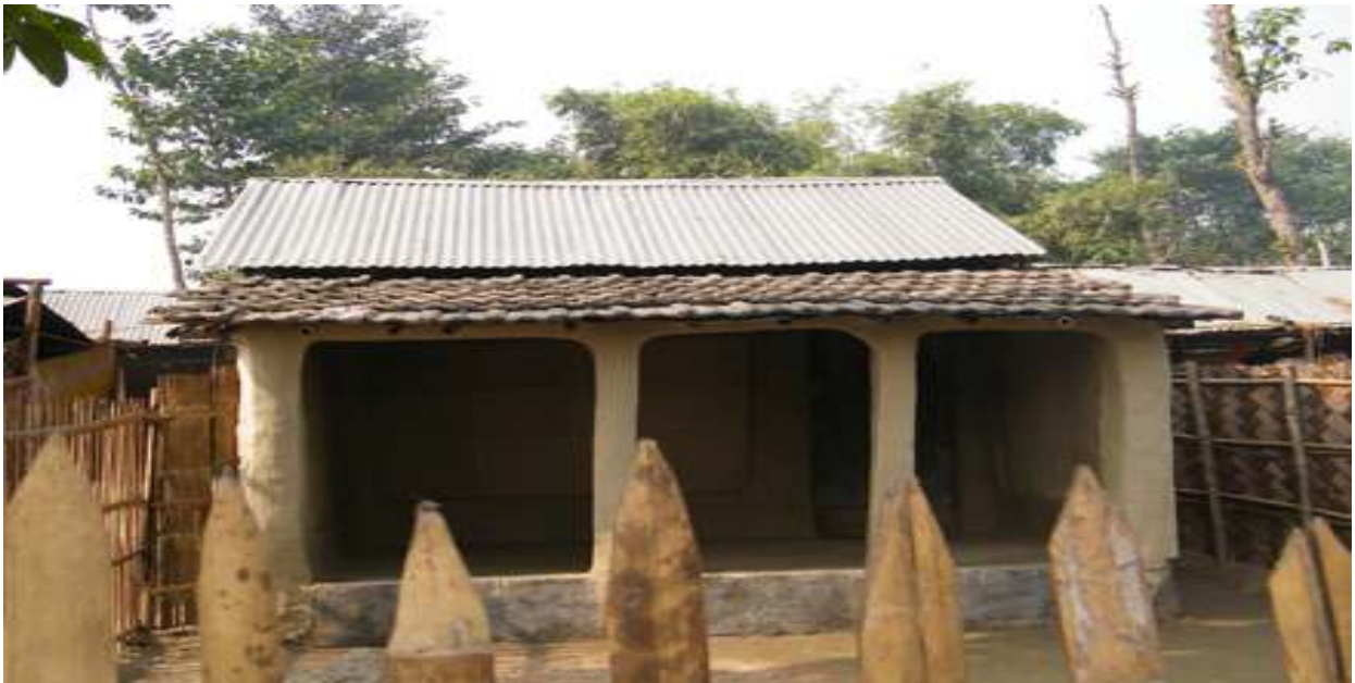
Fig 3.11 A fusion house: tile-roof verandah; GI-sheet roof for main house, mud walls, bamboo roof structure. A lot of the materials are recycled materials retrieved from the old damaged house.
