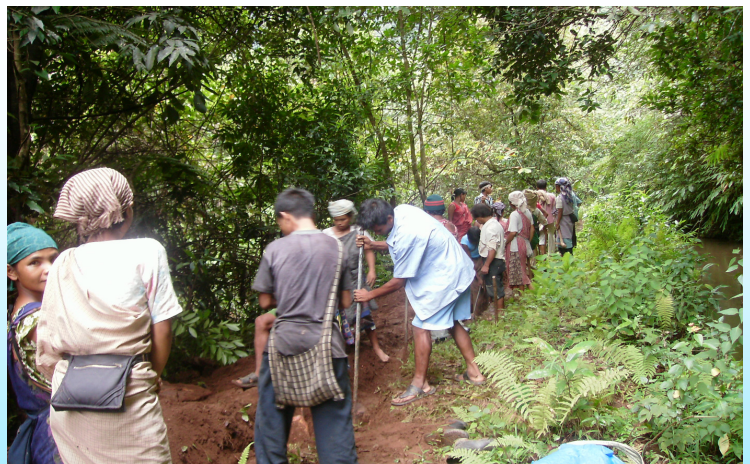
The villagers excavating soil for laying of pipelines
