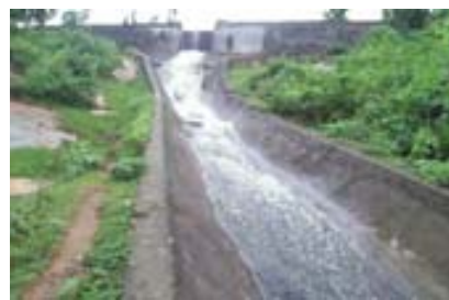
The 500-metre canal
