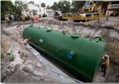
Stormwater Capture & Reuse Tanks
