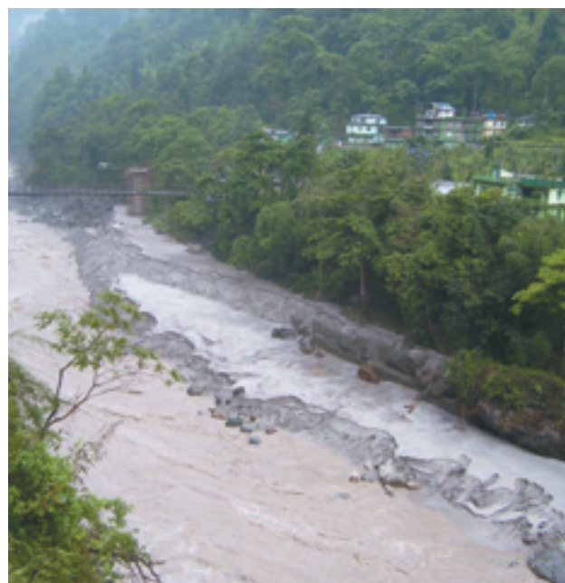
Silt accumulation upstream of Teesta V Dam, 2008. Siltation is a serious issue as it affects the performance and life of a project, and also deprives downstream plains of nutrients that have been the source of their fertility. Photo: River Basin Friends, India
