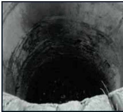
Unused Panchayat Well
