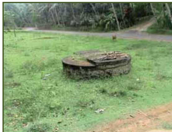
Storage Gallery at Uchakada Pump House
