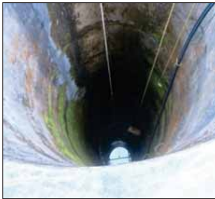
Open well water source
