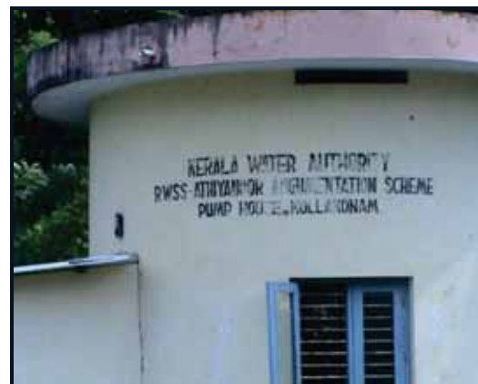
Pump house at Kollamkonam
