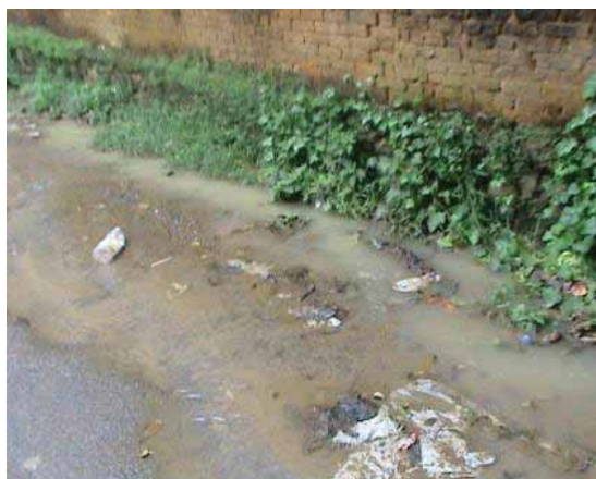
Overflow into the main roads
