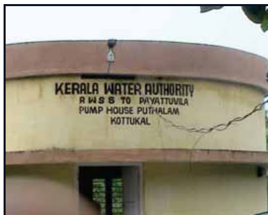
Pump House at Puthalam
