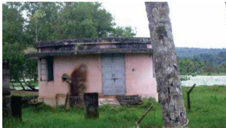
Closed Pump House in Vellayani
