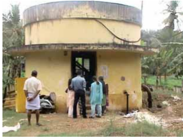
Kakkamoola Pump House
