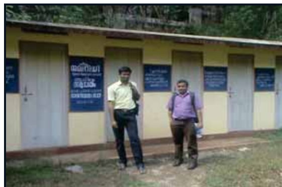
Sanitation facility by Jalanidhi -1
