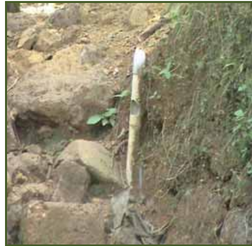
Damaged pipeline
