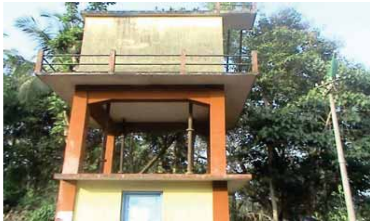
Over Head Tank
