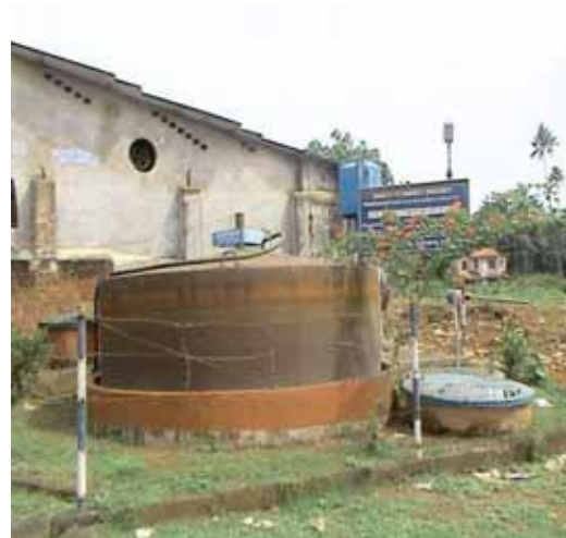
Bio Waste Treatment Plant
