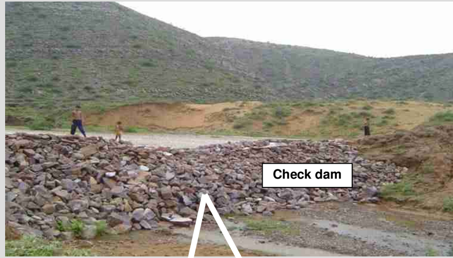
Figure 10 : High nitrate & fluoride levels reduced due to check dam
