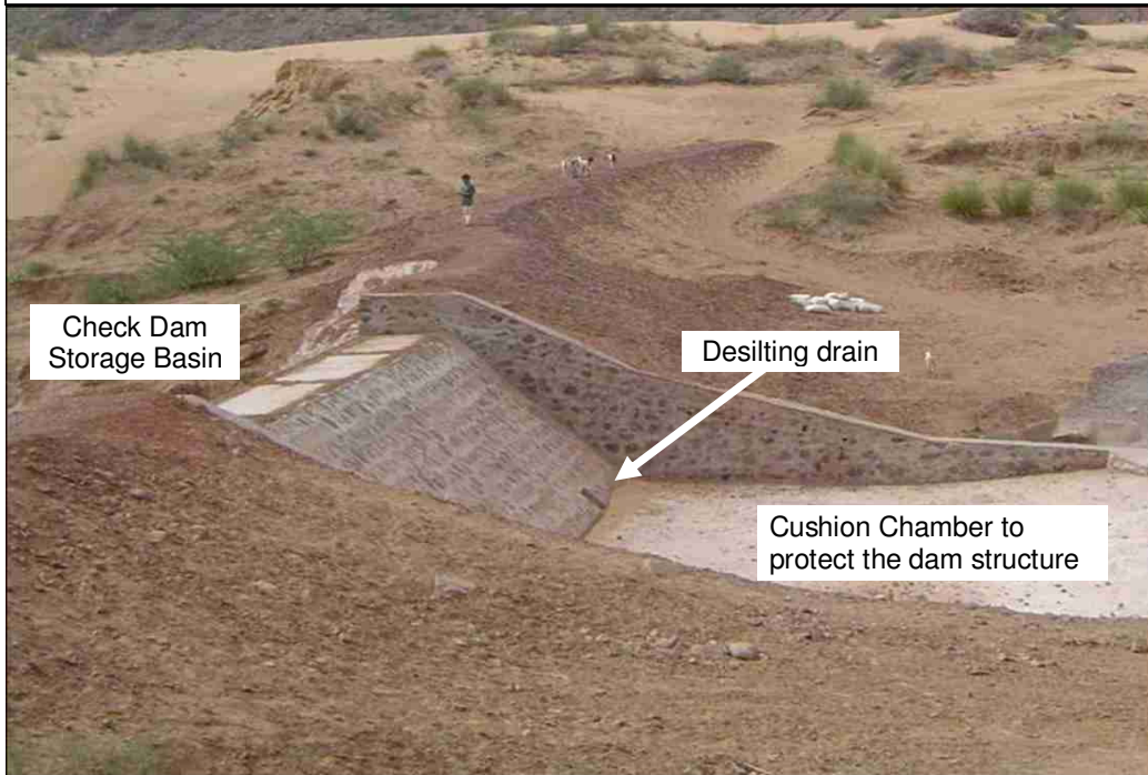
Figure 8 : Ghaghas Masonry Check Dam
