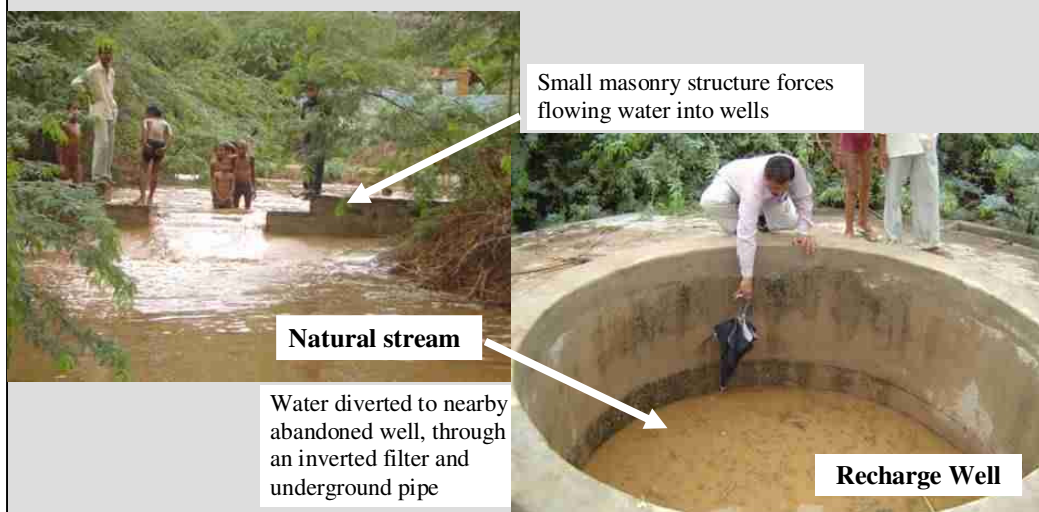
Figure 5: Ground-water Recharging through well in Ghaghas
