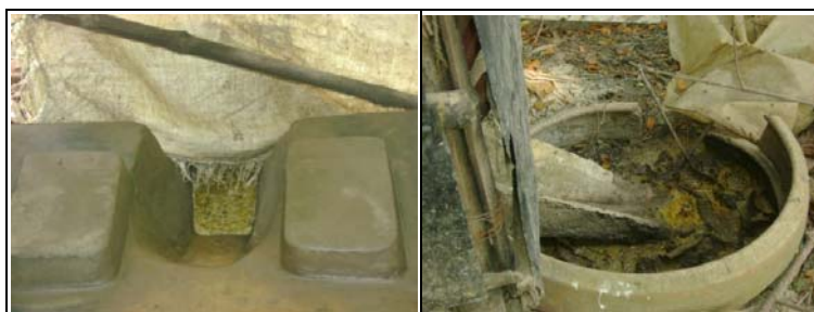
Service latrine in Charmasdigha GP (West Bengal) – Front and Back View
