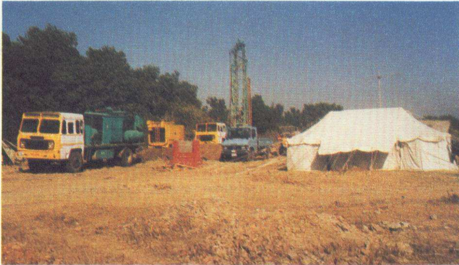
IIIa Drilling of a tubewell in village Ghagwal
