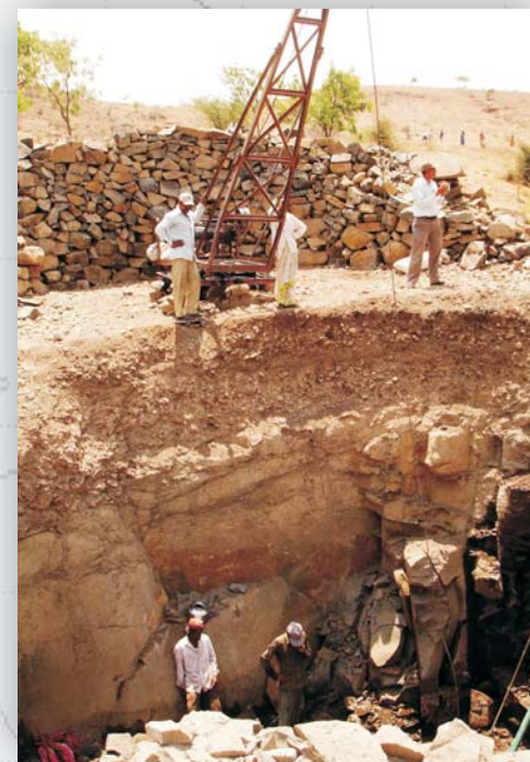
Digging of new dug well in Pondhe
