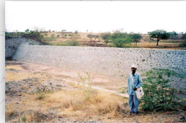
Check dam in Purandar
