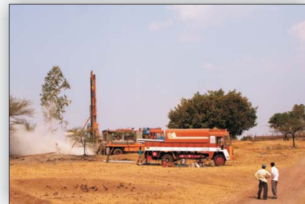
Drilling going on in Pondhe for drinking water supply scheme
