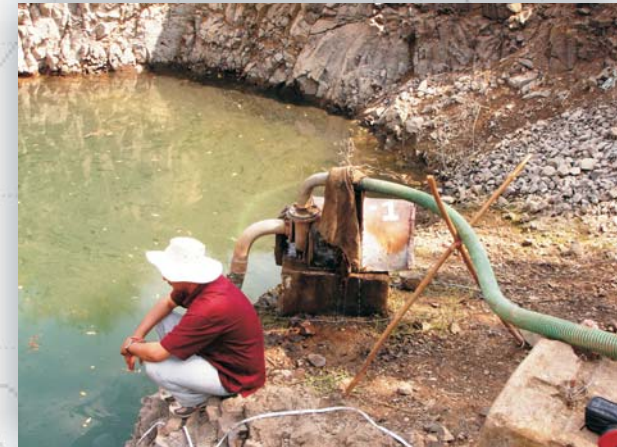
Well with a diesel pump in Naigaon
