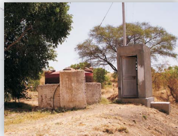
Toilet and a biogas plant constructed by an individual farmer
