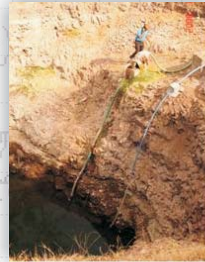
Automatic water level recorder installed in Naigaon well
