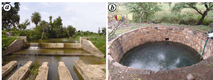
Figure 2. a, Eight such check dams generated 25,000 m 3 surface water-storage capacity; b, Well full of water in a watershed.
