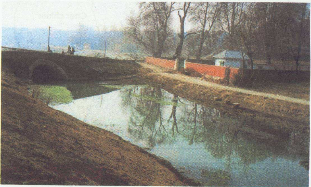
Fig. 2: A view of Telbal Drain at upstream side near the entry point to Dal - Nagin Lake
