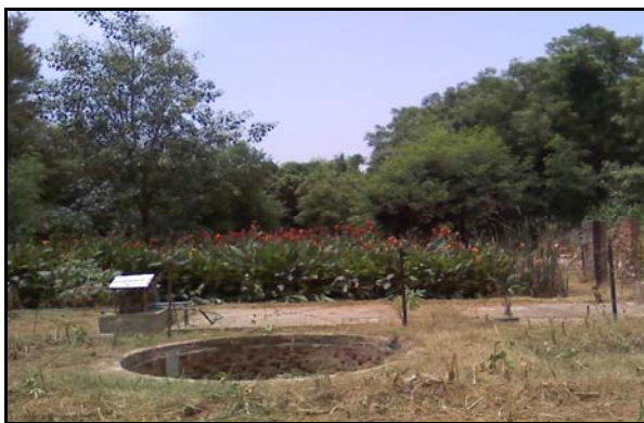
Figure 2: IIT-Delhi WWT R&D Plant
