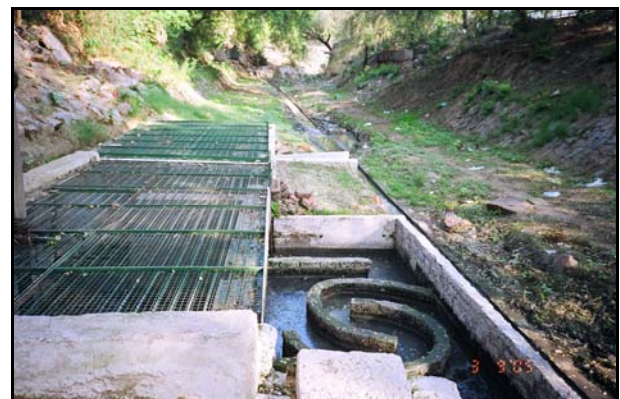
Figure 3: Vasant Vihar WWT Plant
