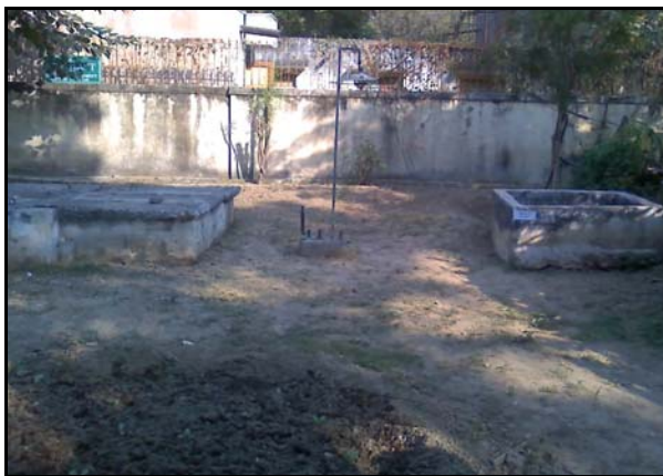
Figure 4: Bio-Gas Plant at AIWC, Delhi.
